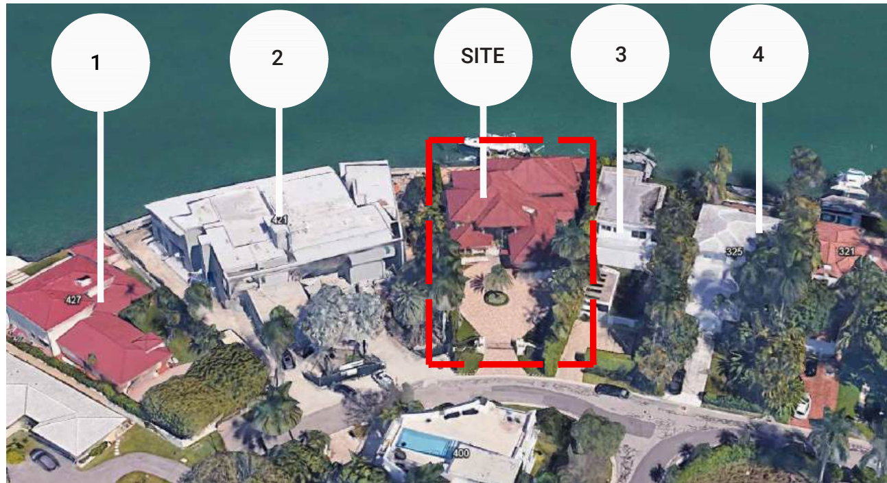
AERIAL PHOTOGRAPH - FRONT OF RESIDENCE
