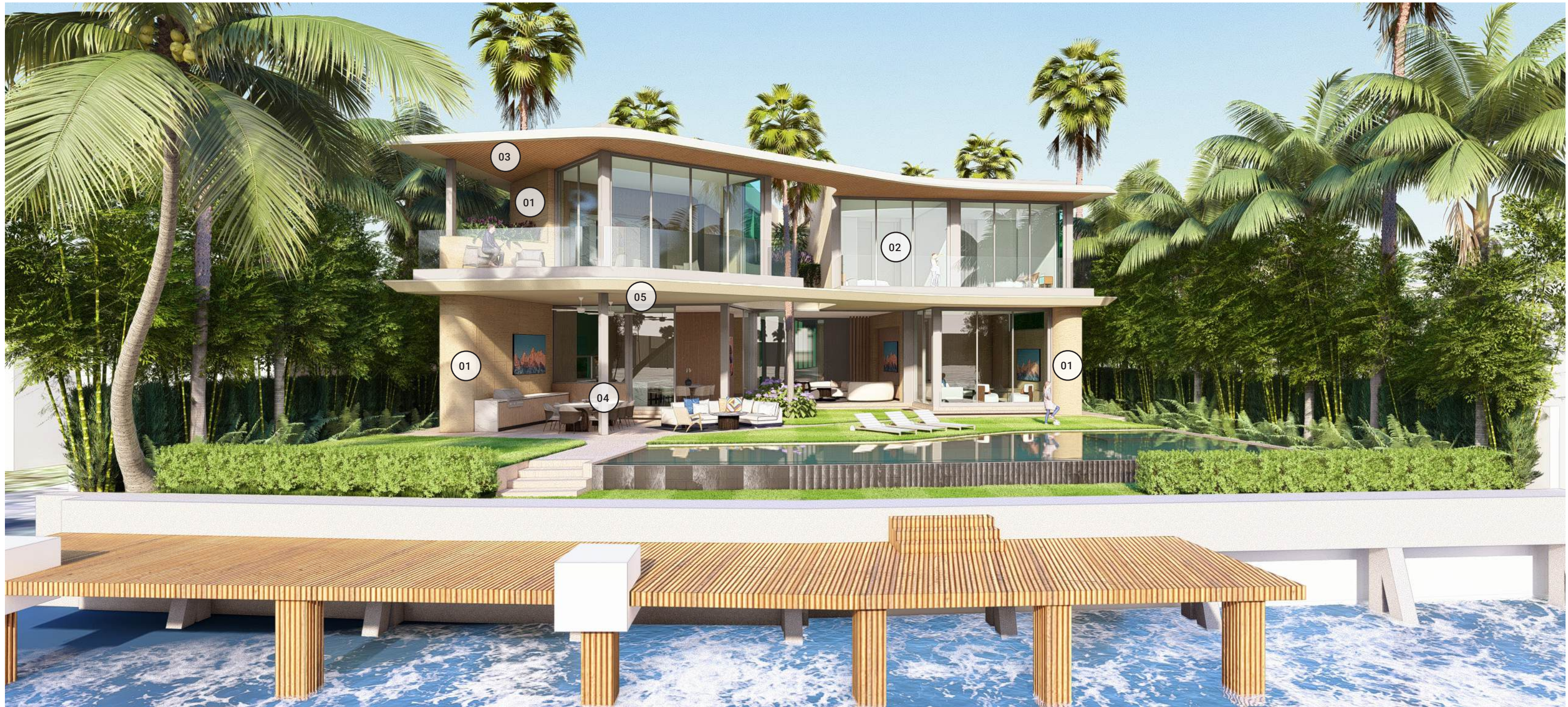
REAR OVERALL_FROM BAY LOOKING WEST
