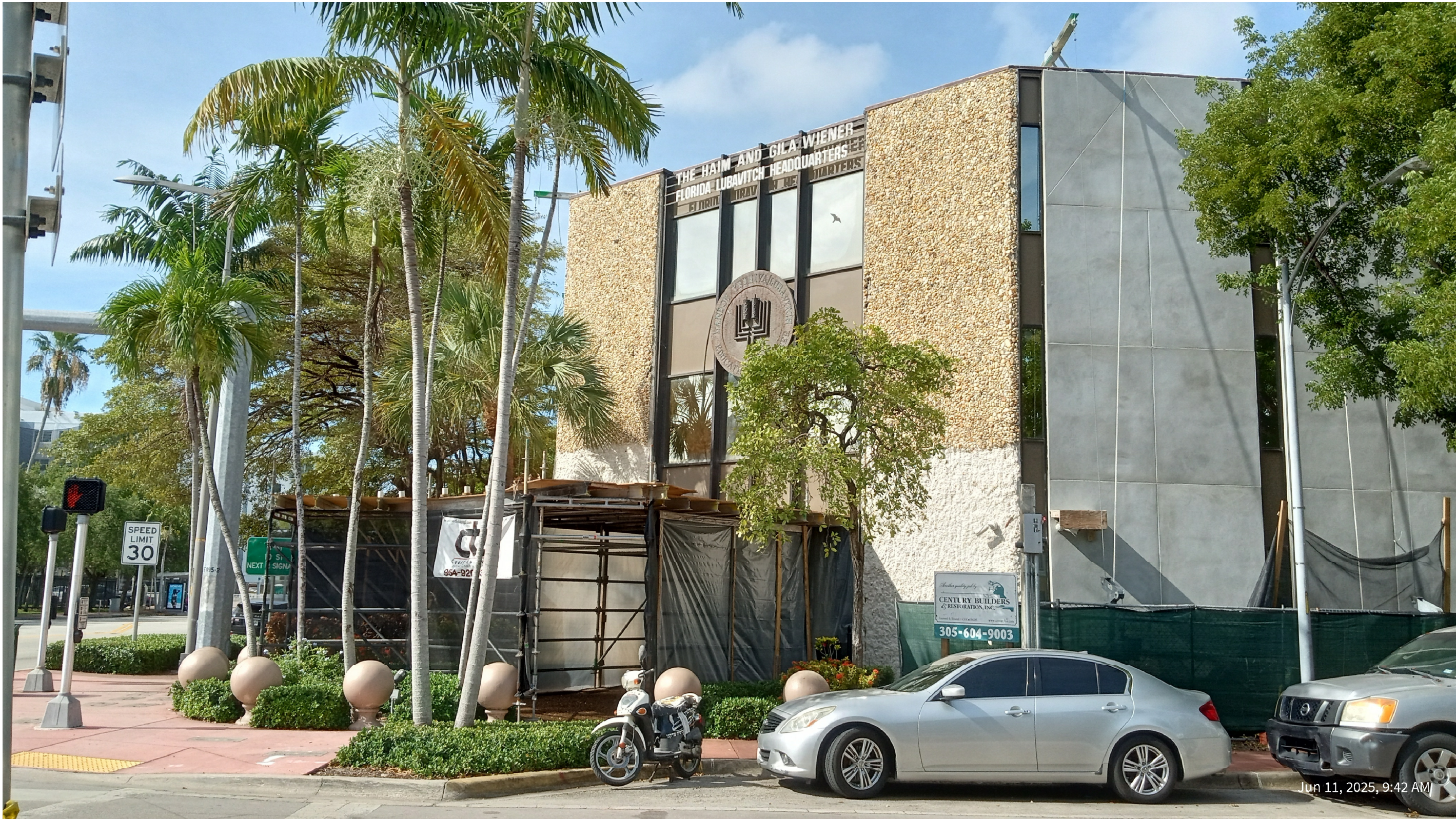
CORNER EXISTING FACADE
