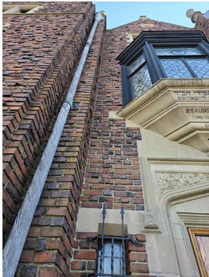
PRECAST STONE MOULDING
