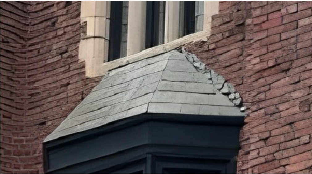
EXISTING SLAT ROOF
