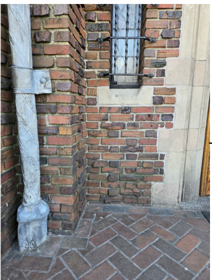
PRECAST STONE MOULDING AND BRICK
