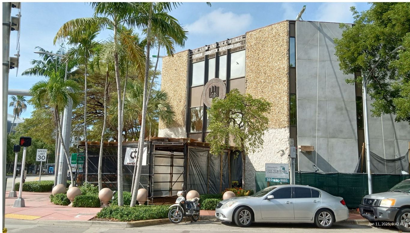
1) CORNER EXISTING FACADE
