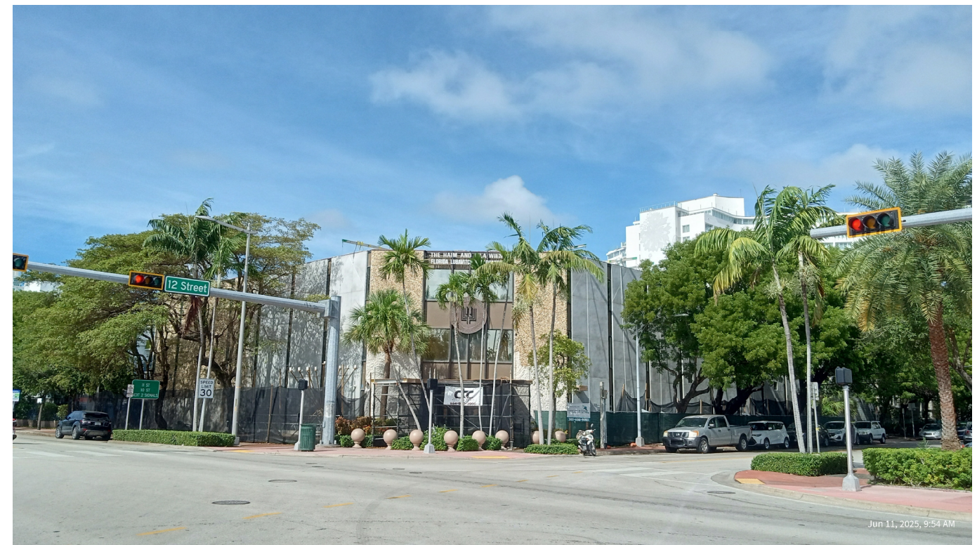
2) CORNER FACADE VIEW FROM ALTON ROAD
