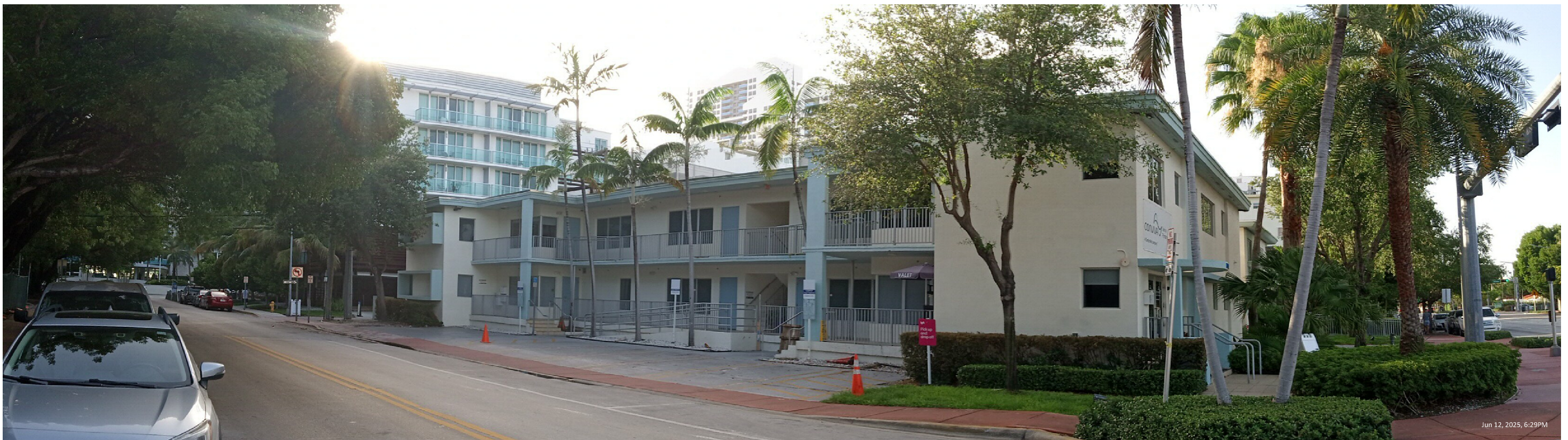
CONTEXTURAL PANORAMIC ALONG 12 TH STREET - LOOKING NORTH
