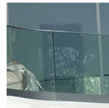
GL2 IMPACT GLASS HANDRAIL- CLEAR, RADIUSED CORNERS
