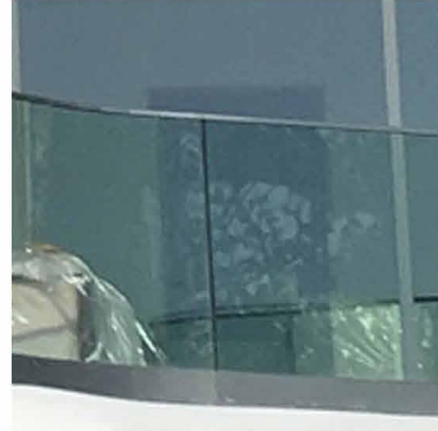
GL2 IMPACT GLASS HANDRAIL- CLEAR, RADIUSED CORNERS
