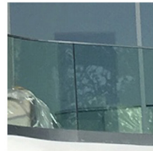
GL2 IMPACT GLASS HANDRAIL - CLEAR, RADIUSED CORNERS
