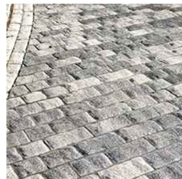
Permeable Paver Type Alternative (drive surface only)
