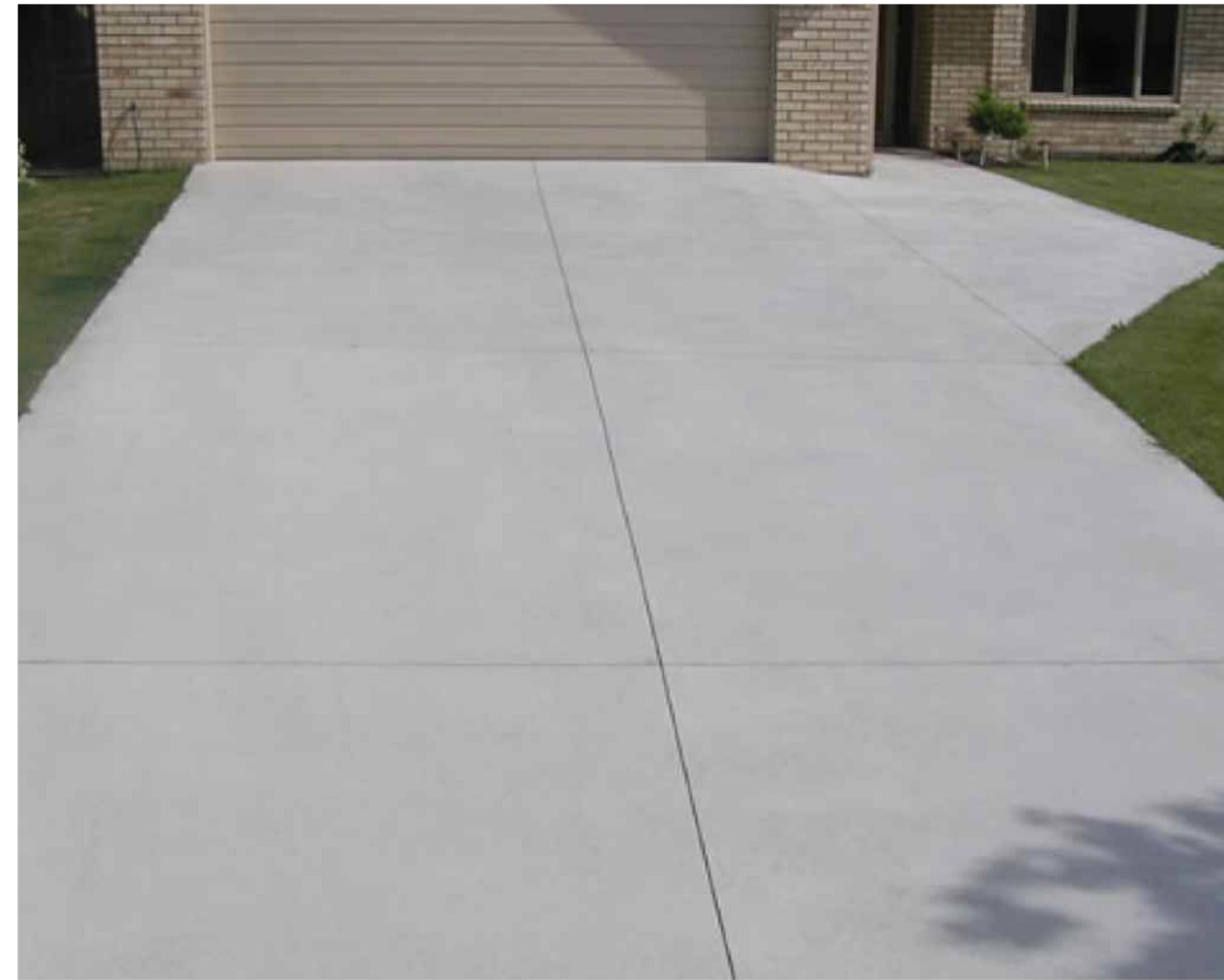
BRUSHED CONCRETE EXTERIOR
