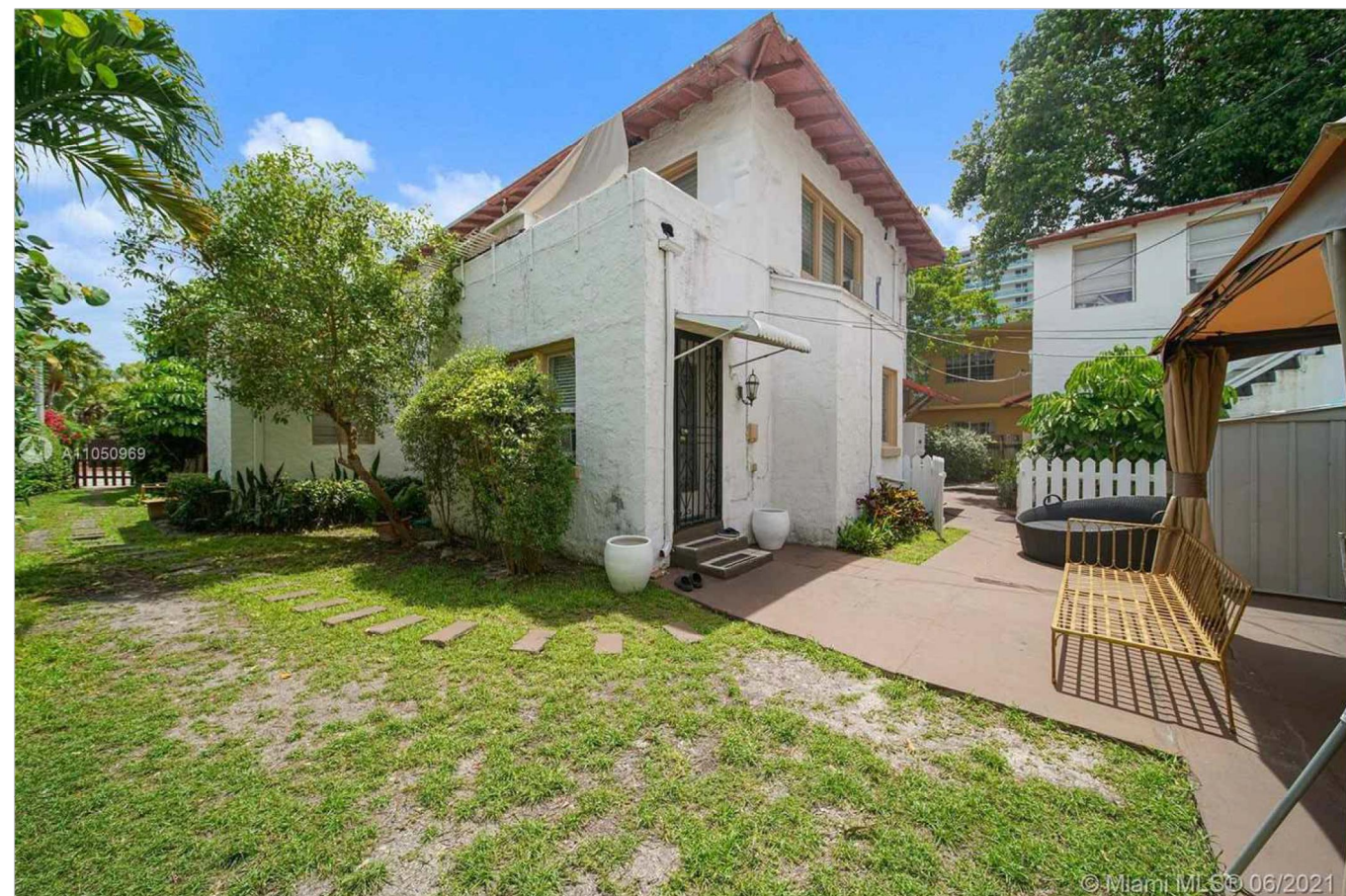
REAR YARD EXISTING SCALE N.T.S
