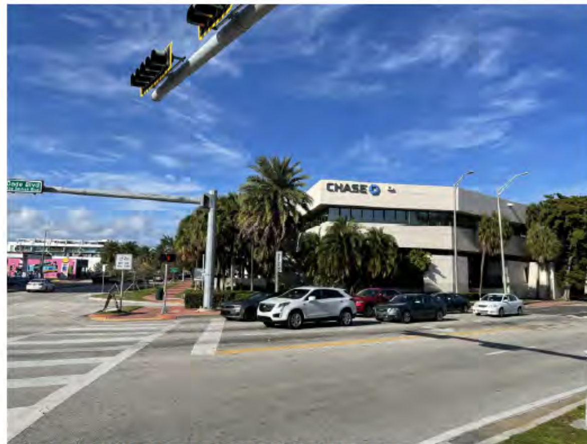
04 ALTON ROAD / DADE BLVD LOOKING NORTH AT 1801 ALTON ROAD
