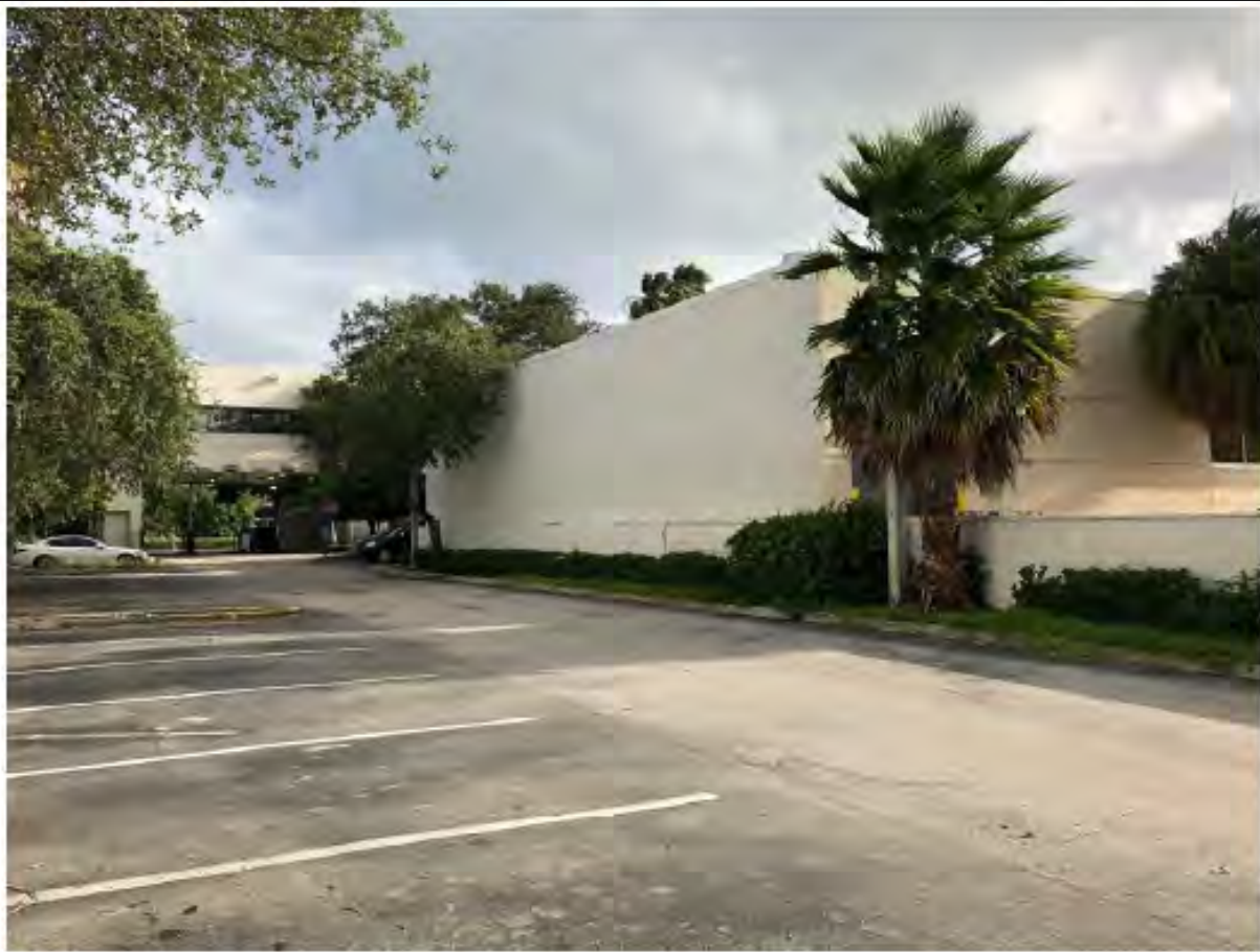
13 EXISTING PARKING LOOKING SW
