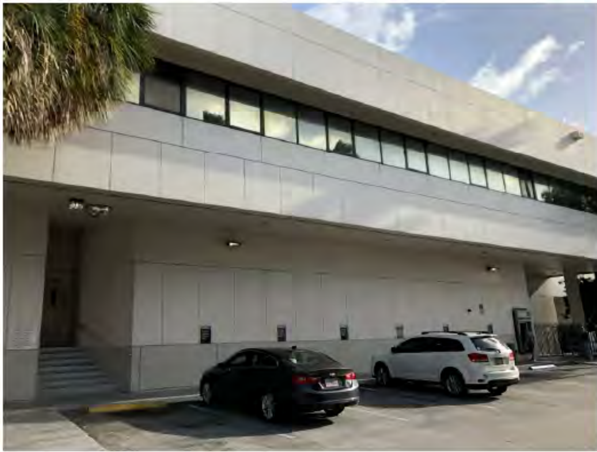
09 EXISTING PARKING LOOKING SW
