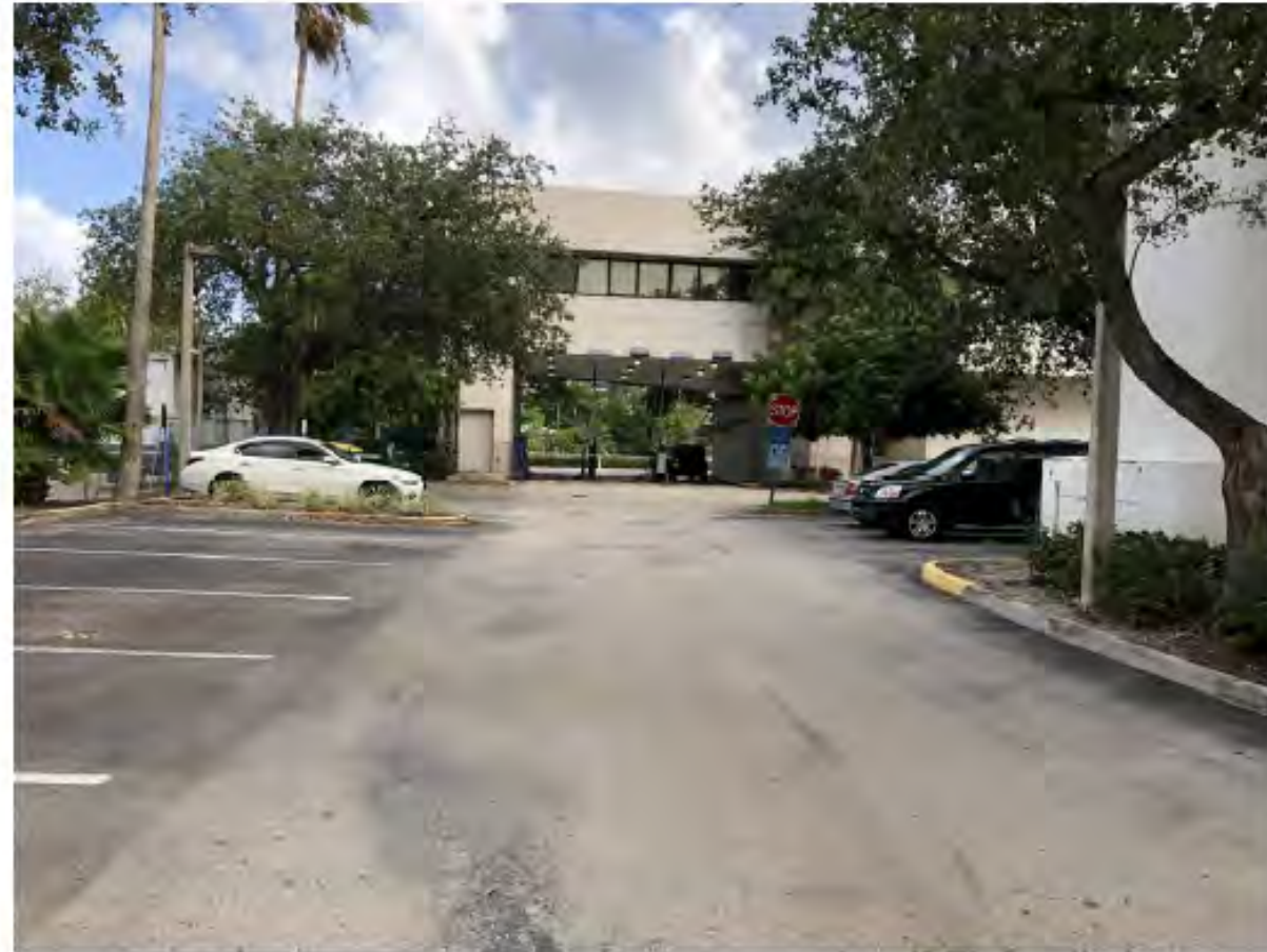
12 EXISTING PARKING LOT LOOKING SOUTH
