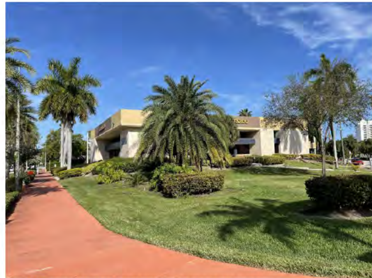
24 ALTON ROAD / 19TH STREET LOOKING NORTH AT WELLS FARGO
