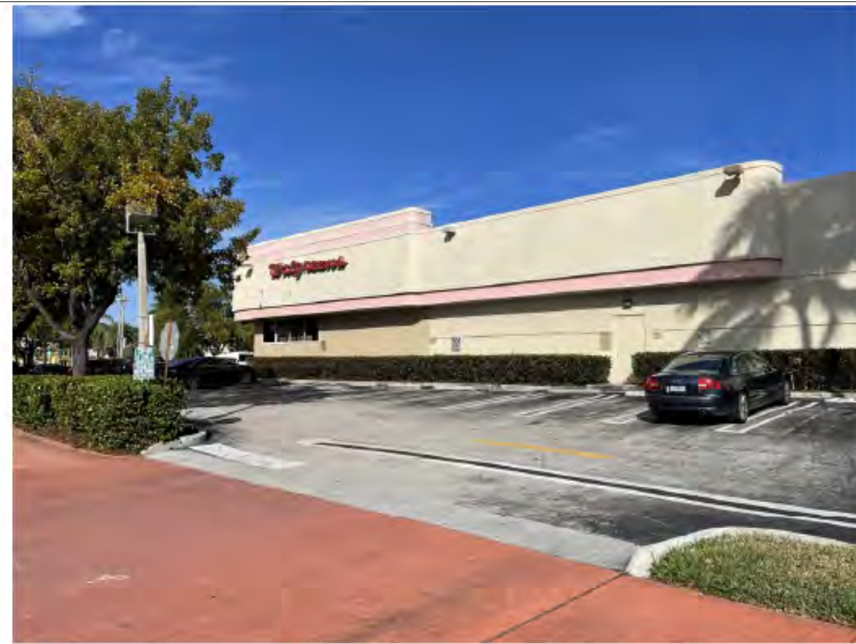
22 ALTON ROAD LOOKING NORTH EAST AT WALGREENS
