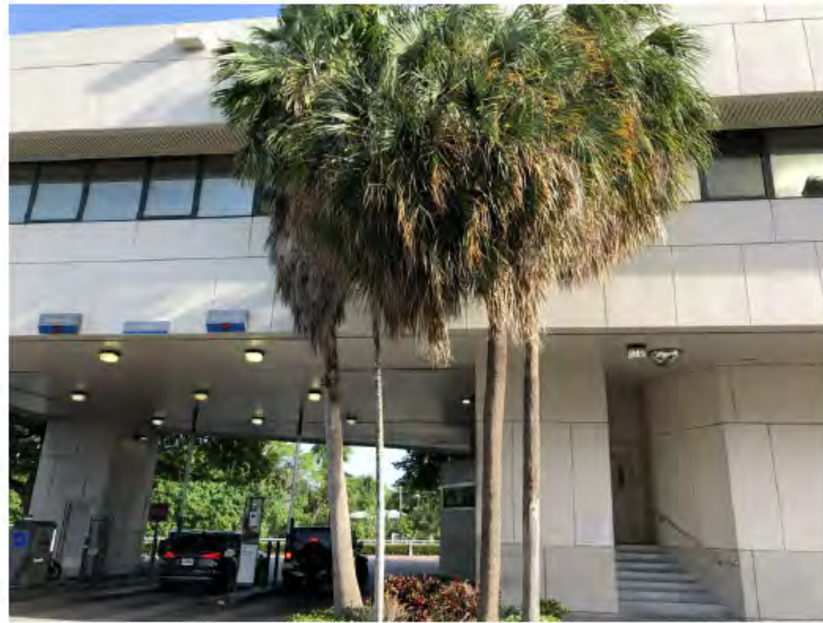
10 EXISTING PARKING LOOKING SOUTH
