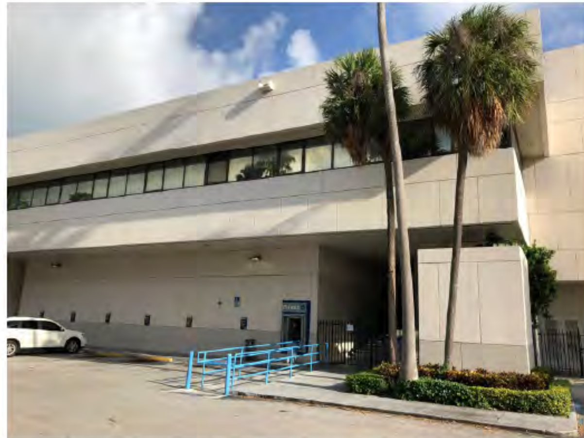
08 EXISTING PARKING LOT LOOKING SOUTH
