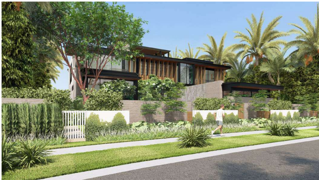
FRONT OVERALL _ FROM DIDILO DR. [LOOKING NORTHWEST]
