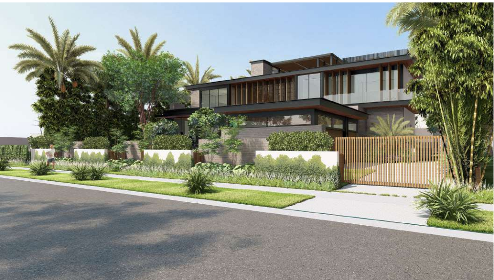
FRONT OVERALL _ FROM DIDILO DR. [LOOKING SOUTHWEST]
