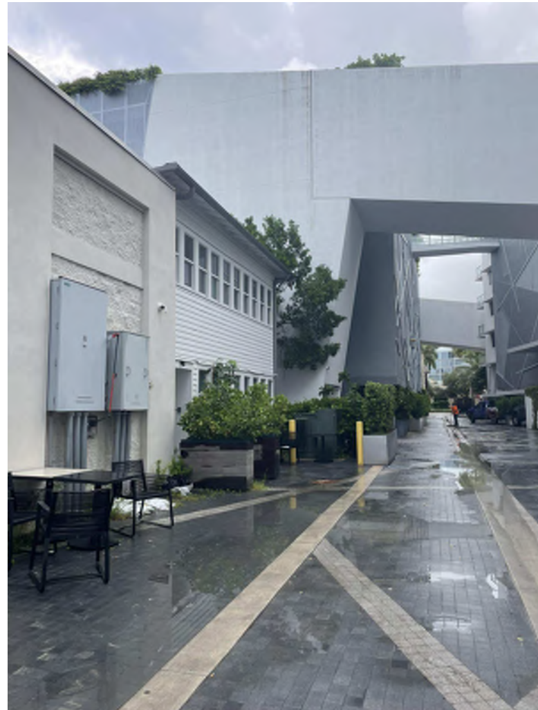
PHOTO A: REAR ALLEYWAY
