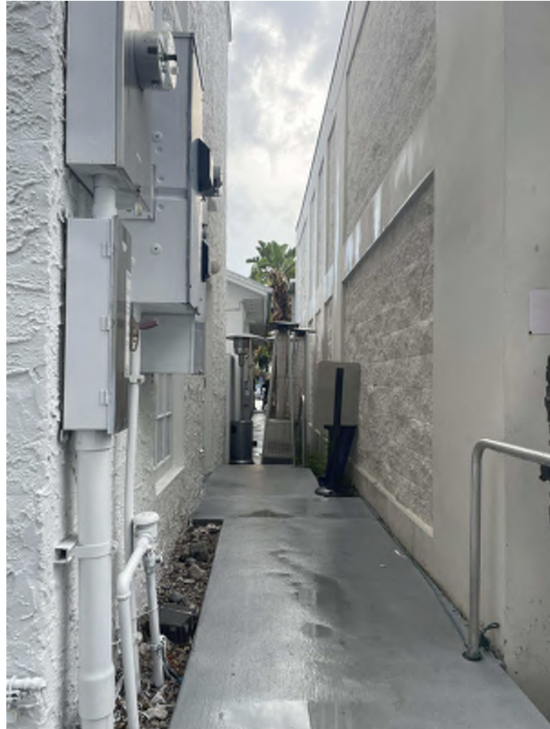
PHOTO C: LEFT SIDE OF BUILDING
