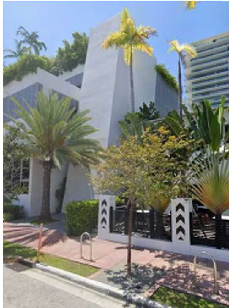
PHOTO A: BUILDING ON PLAN WEST
