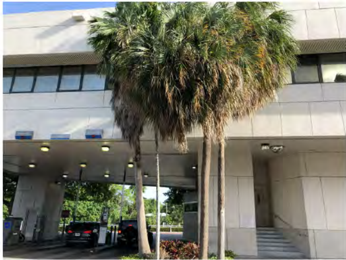
10 EXISTING PARKING LOOKING SOUTH
