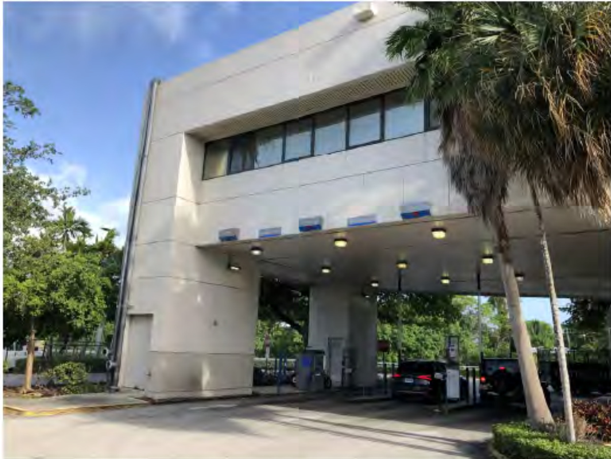
11 EXISTING PARKING LOOKING SOUTHEAST
