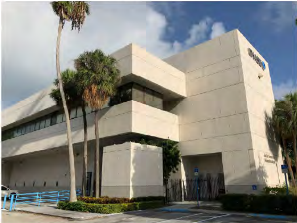
07 ALTON ROAD LOOKING SOUTHEAST
