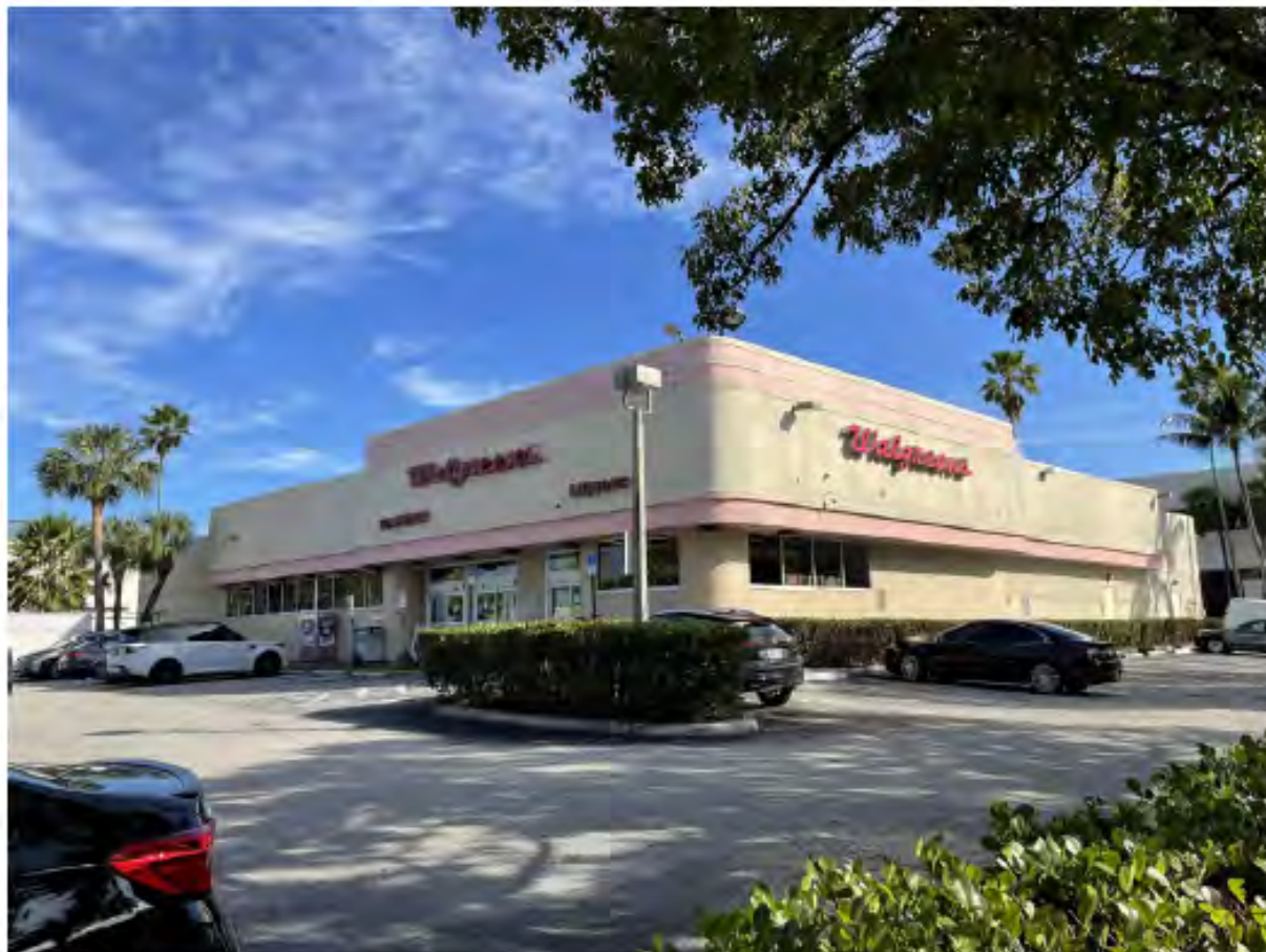
23 ALTON ROAD / 19TH STREET LOOKING SOUTHEAST AT WALGREENS
