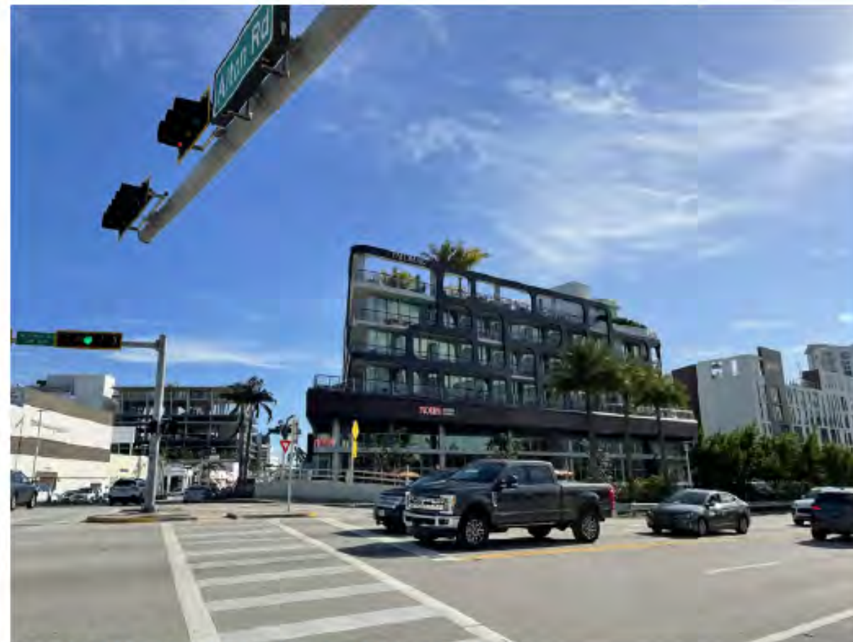
20 ALTON RD / DADE BLVD LOOKING SOUTH AT THE PALOMAR
