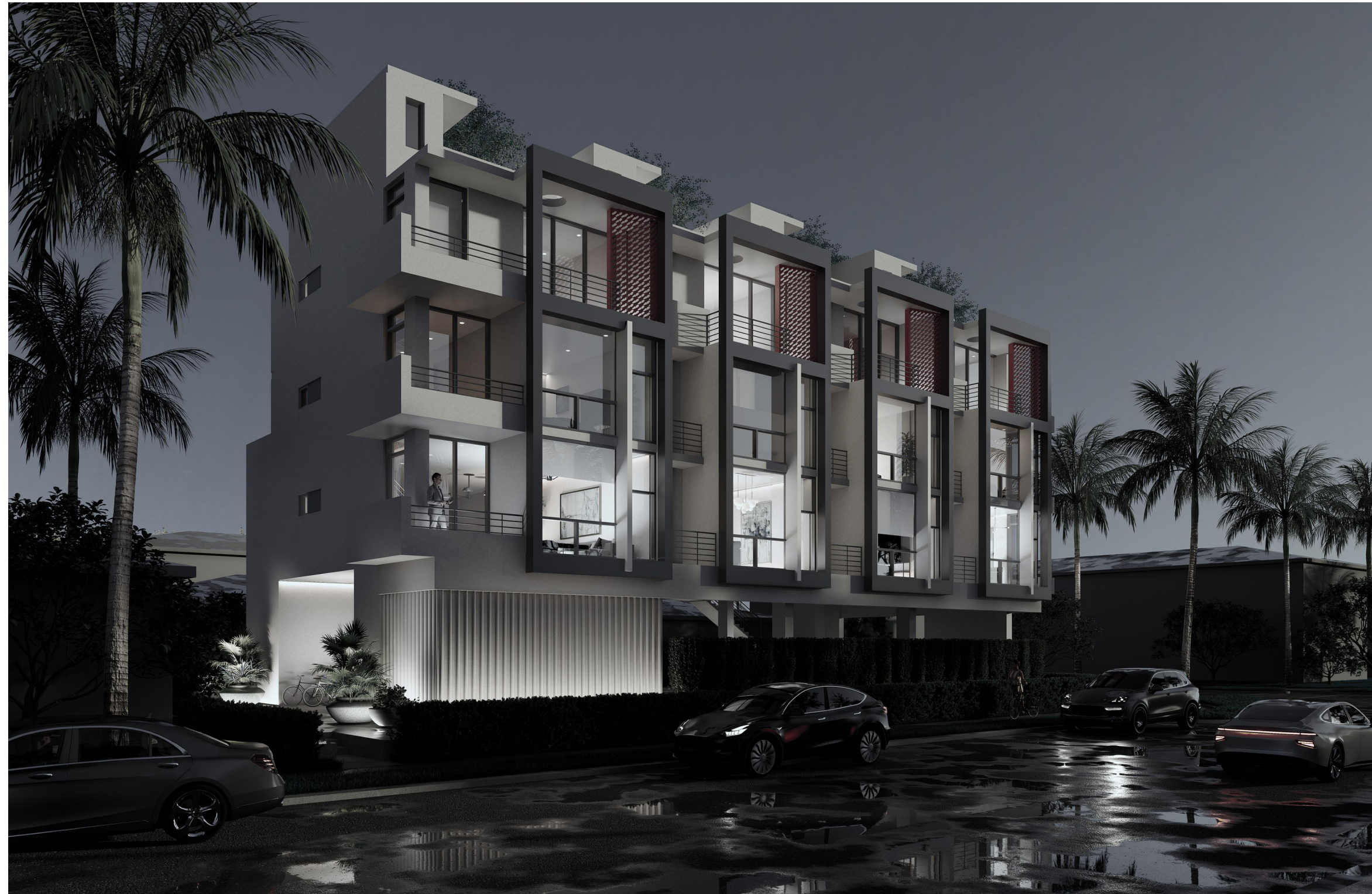
NIGHT VIEW FROM NORTHWEST
