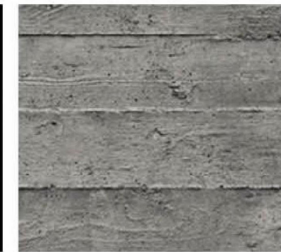
C1 BOARD CONCRETE
