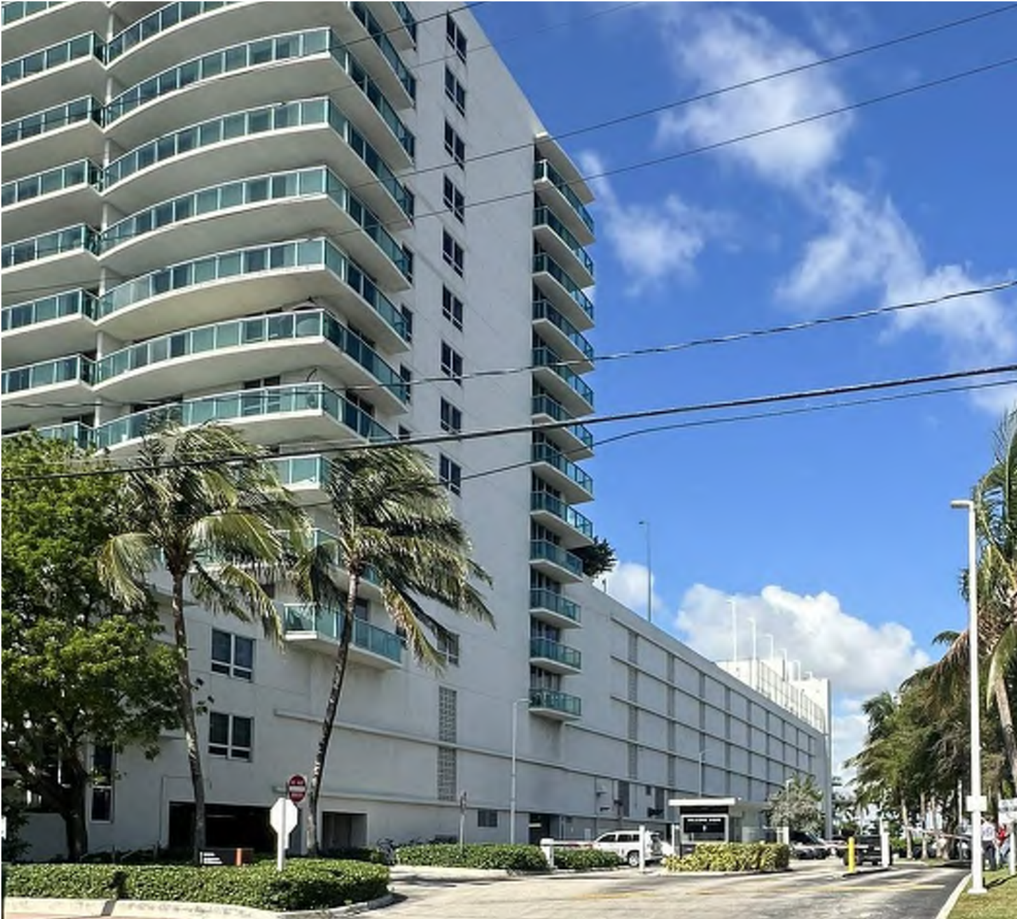
Existing Bay Road View
