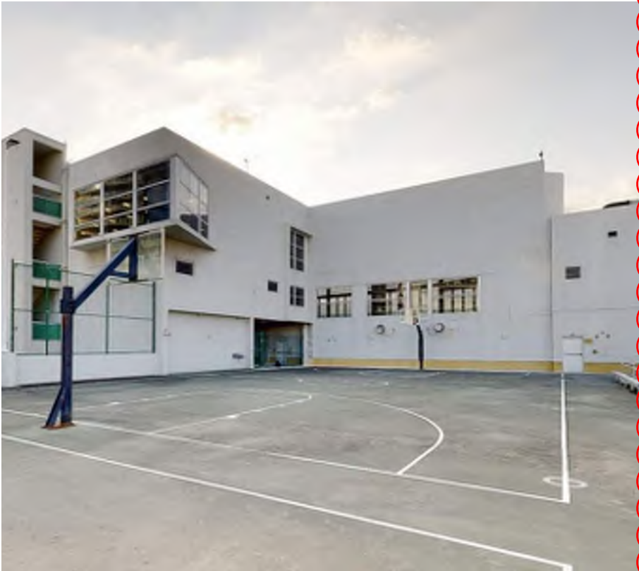
Existing Basketball Court
