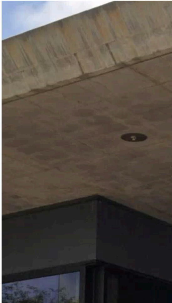
EXISTING OFF FORM CONCRETE
