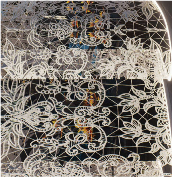
NEW LASER CUT WHITE POWDERCOATED ALUMINUM SCREENS
