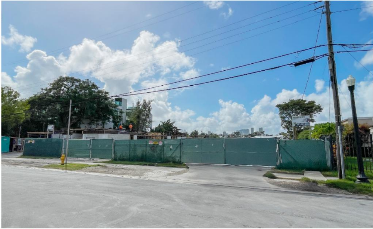
1 320 W DI LIDO DRIVE CONSTRUCTION IN PROGRESS
