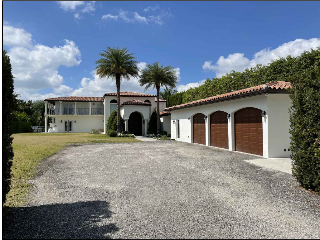
E1 - 6470 ALLISON RD - VIEW TO FRONT (EXISTING STRUCTURE)
