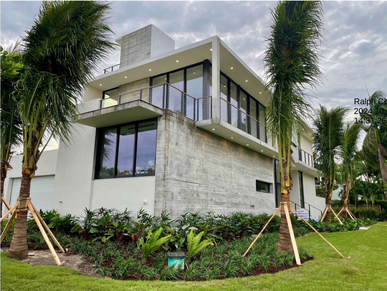
VIEW OF NORTH EAST CORNER
