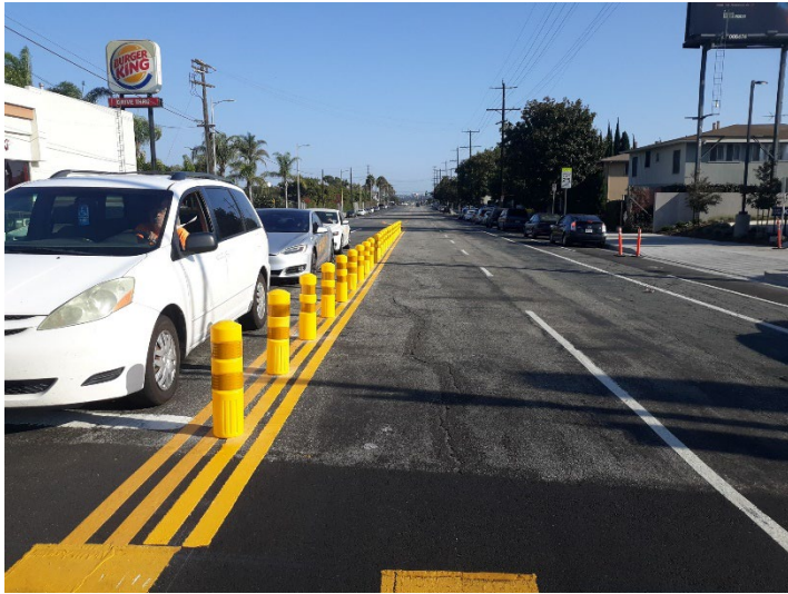
Example of K71 Bollards in the Median
