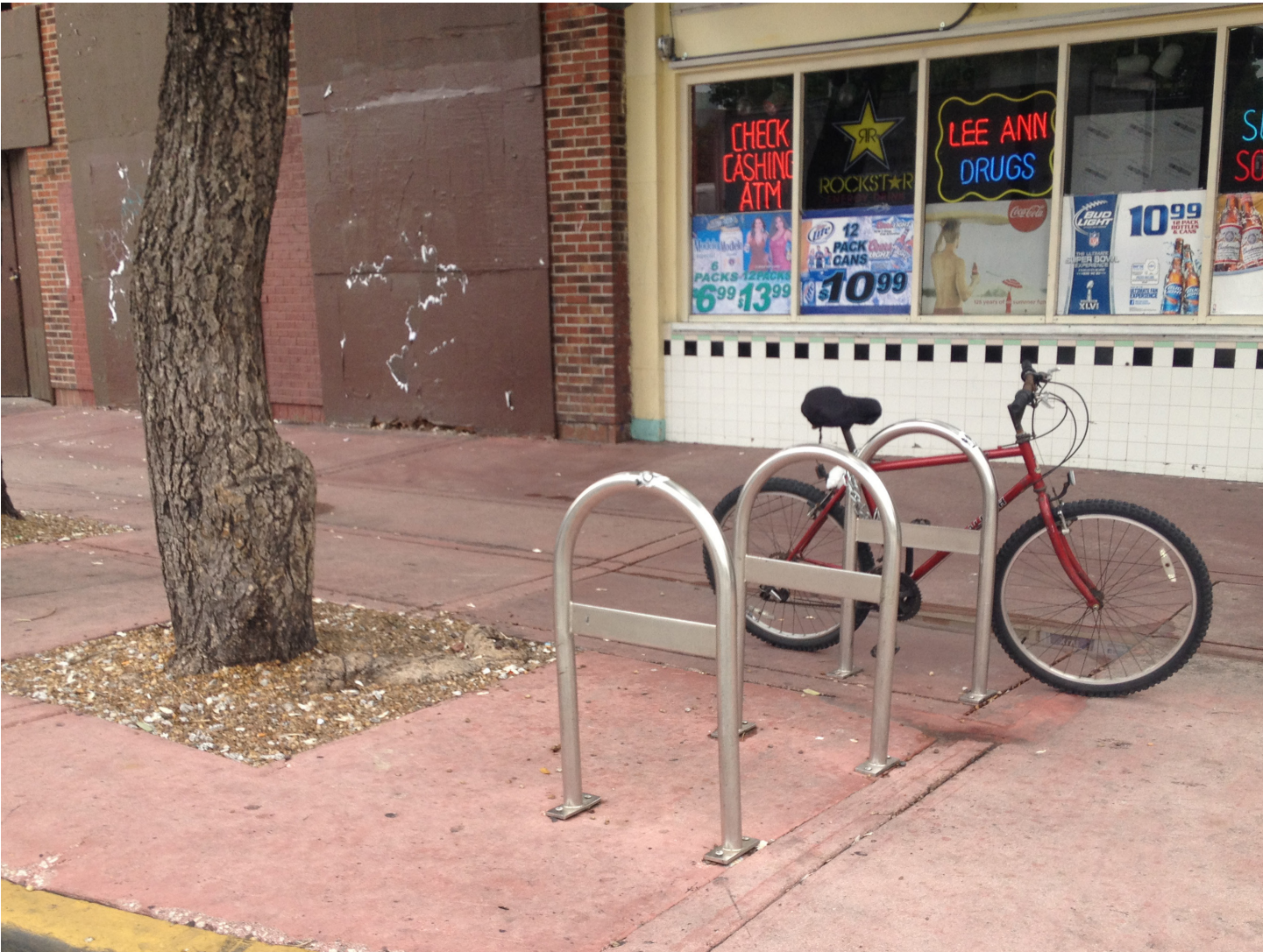
The above bicycle parking is well-spaced, properly oriented parallel to the curb, and a safe distance from the tree and the curb. See page 126 of the Street Design Guide for additional information.
