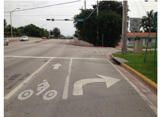
This northbound only Alton Road bicycle lane terminates abruptly at Chase Avenue.
