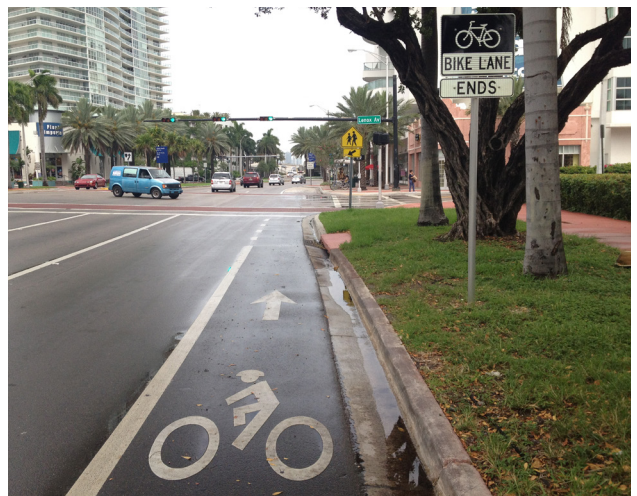
New bicycle lanes along 5th St. improve conditions for skilled bicyclists. However, the eastbound lane ends suddenly at Lenox Avenue, and without indication for how cyclists should continue to navigate.
