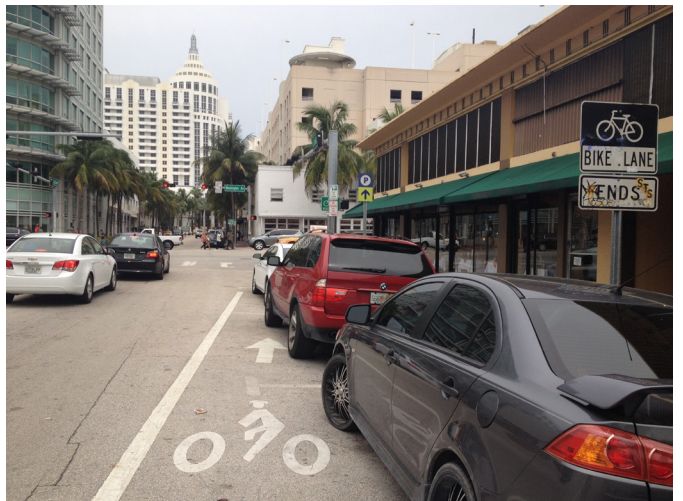
The eastern terminus of the 16th Street bicycle lane directs bicyclists into a row of parked cars.
