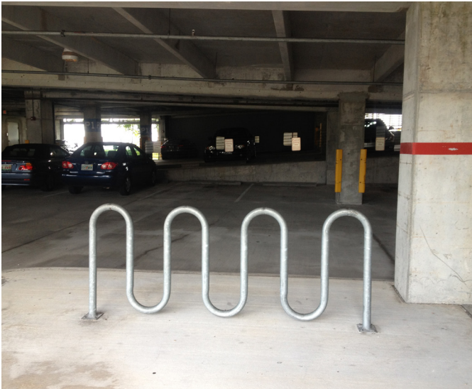
Covered bicycle parking at Mount Sinai's Heart Center's parking garage on Meridian Avenue/West 48th Street.
