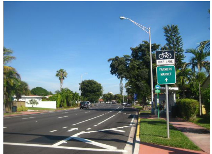
Existing bike lanes on 71 st street.
