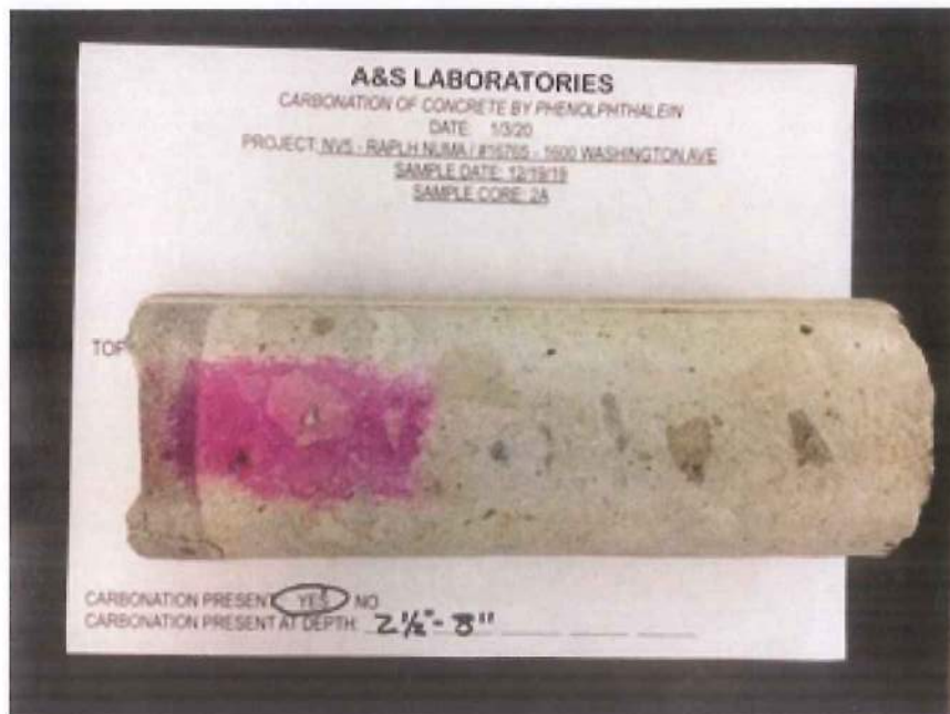
Figure 9: Photograph Core Sample No. 2A: Level 1 Column
