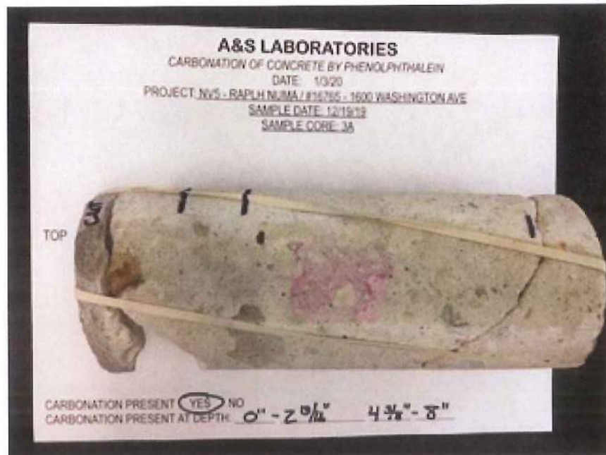
Figure 10: Photograph Core Sample No. 3A: Level 1 Column
