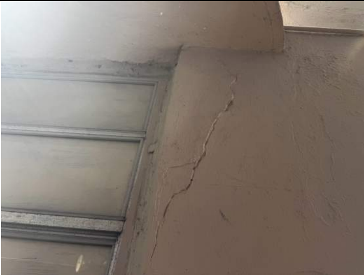
Concrete cracking
