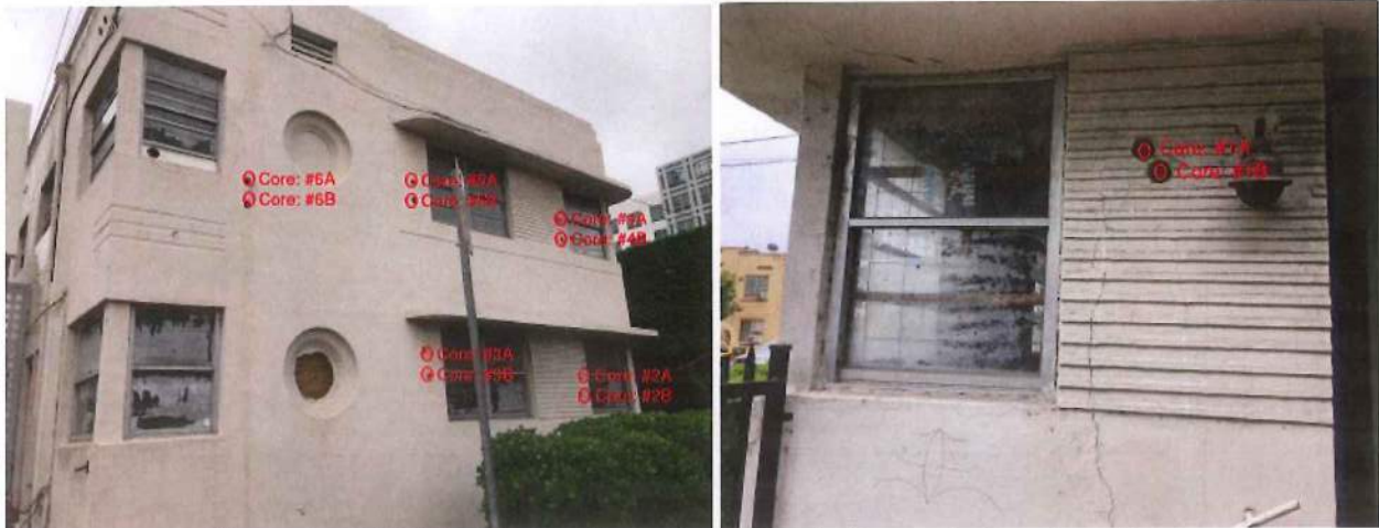
Figure 1: 1600 Washington Ave. - Approximate Concrete Core Locations
