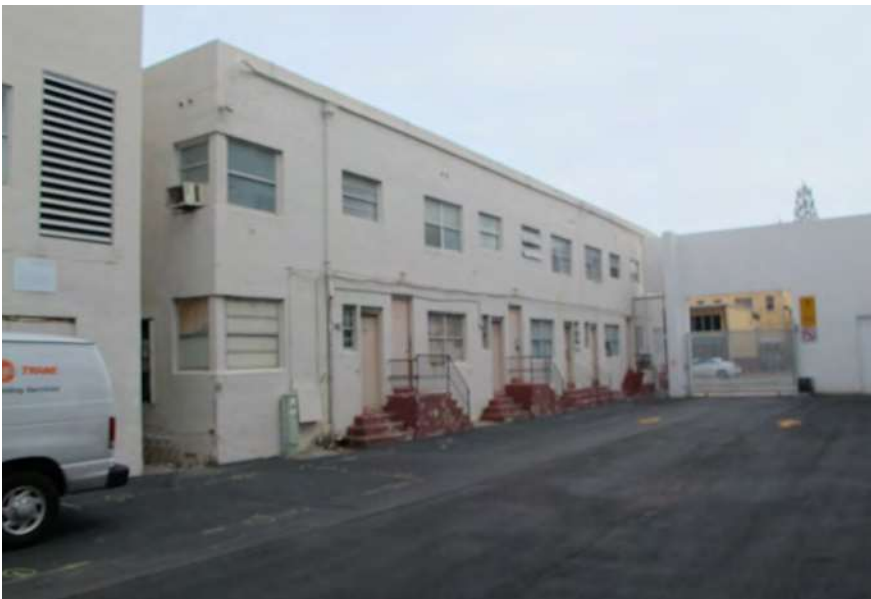
West facade of Laurel Apartments and the 420 Garage service yard View looking south.
