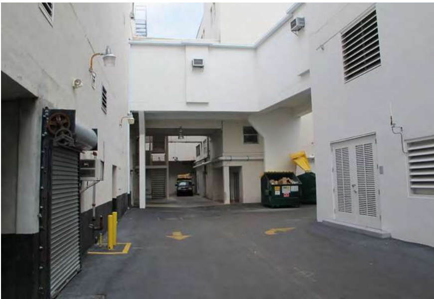
Alley way running between the 420 Garage and the Mercantile National Bank Building. View looking east.
