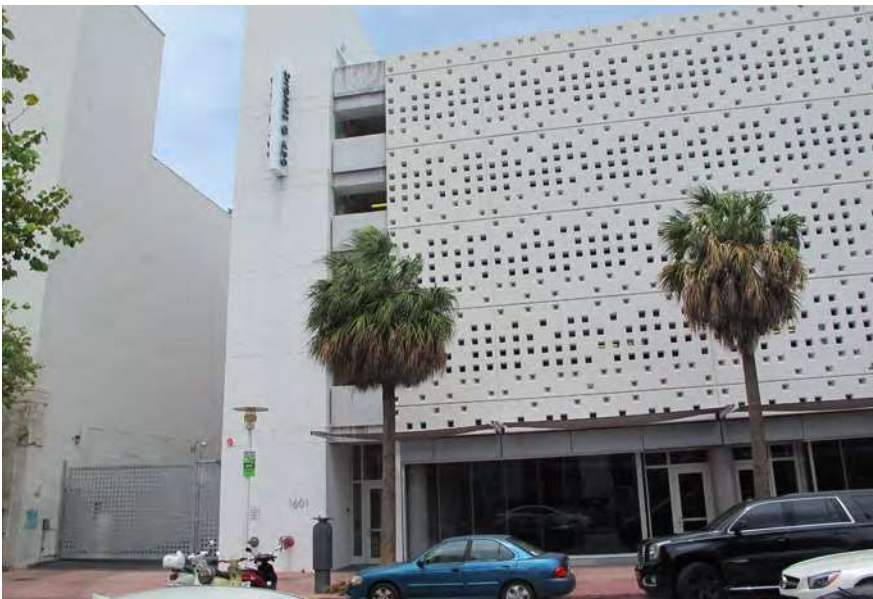
Drexel Avenue Lobby entrance to 420 Garage
