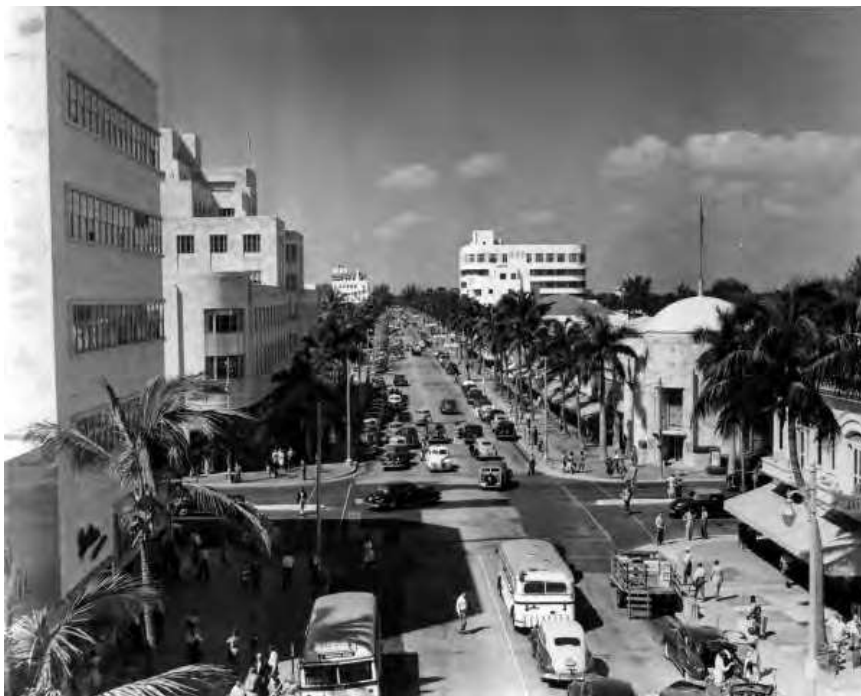
top: Aerial view of the Lincoln Road & Washington Avenue Intersection. 1939. Florida Photographic Collection. BIB Call no. WE240
