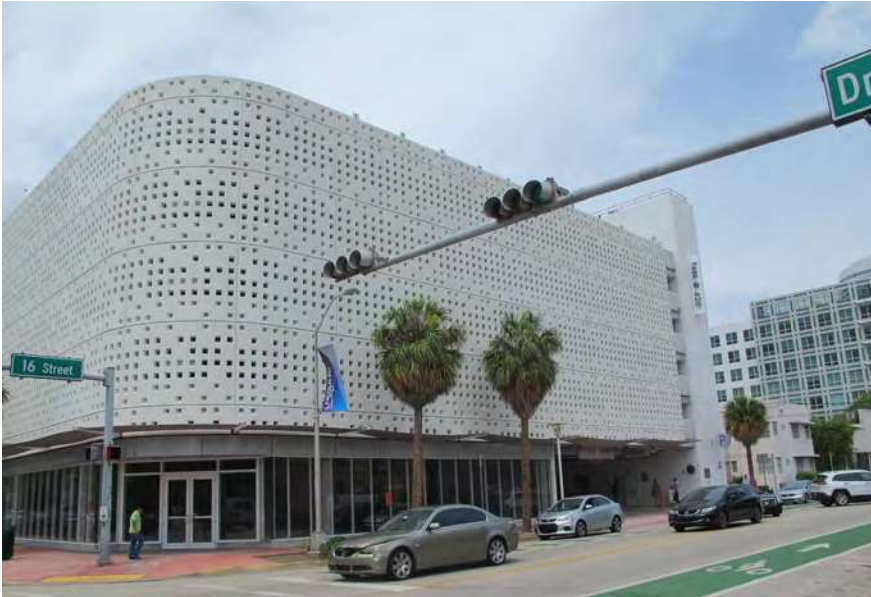
Drexel Avenue and 16th Street corner Frontage View Looking North East
