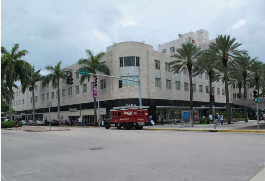
Mercantile National Bank Building Washington Avenue/Lincoln Road corner facade. View looking southwest.
