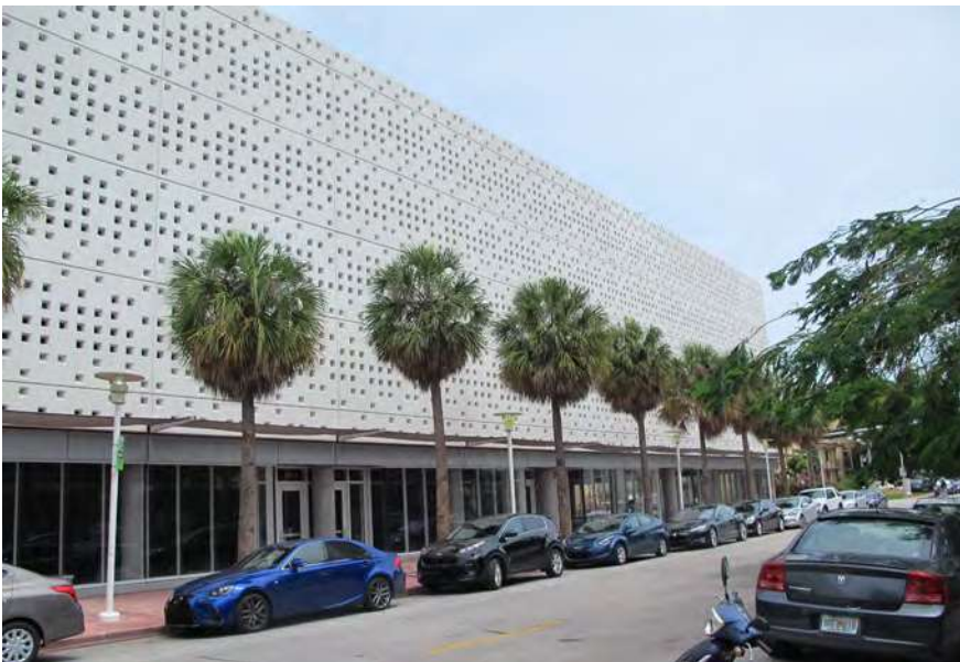
Drexel Avenue Frontage View Looking South
