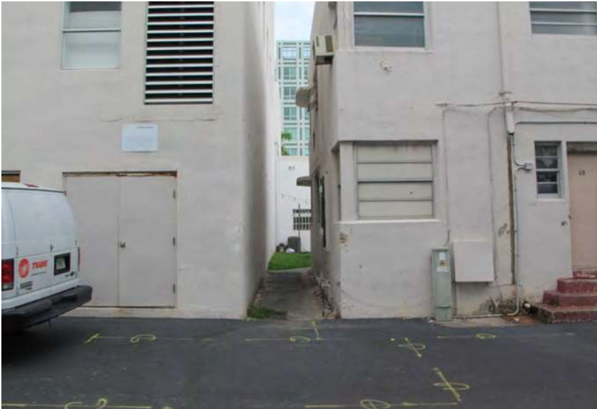
Alley between Laurel Apartments (on right) and Washington Avenue annex of the Mercantile National Bank Building (on left). View looking east.
