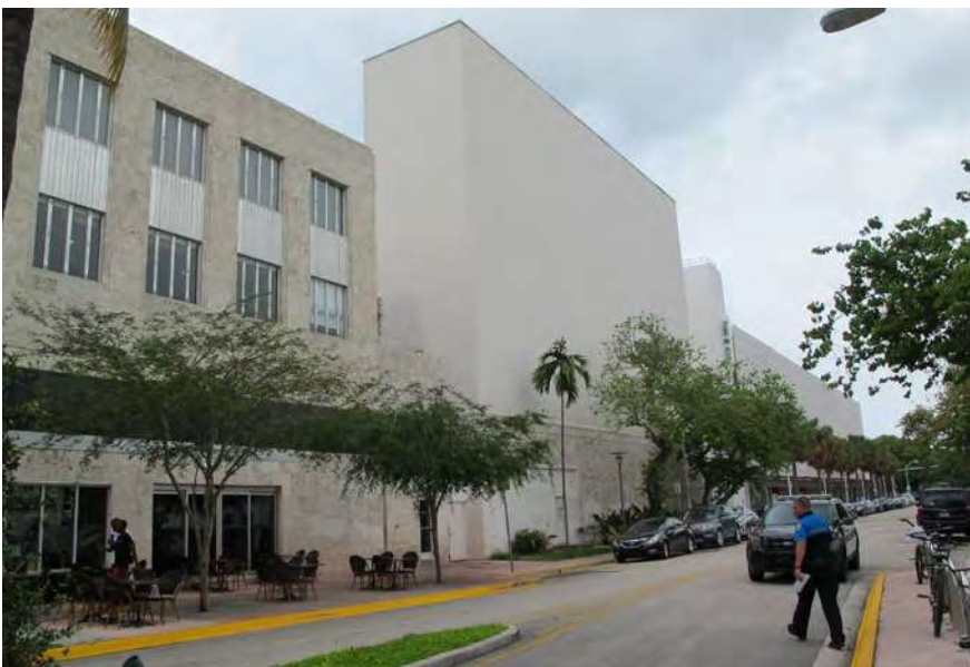
Mercantile National Bank Building Drexel Avenue facade. View looking south.
