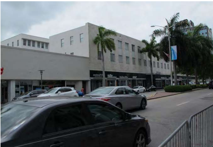
East facade of the Washington Ave- nue Annex to the Mercantile Nation- al Bank Building. View looking Northeast.
