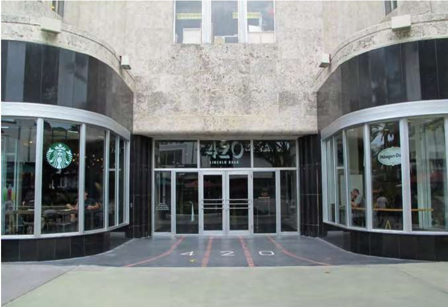
Mercantile National Bank Building Lincoln Road lobby entrance. View looking south
