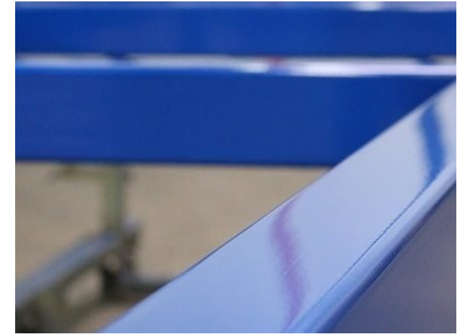
MTL-03: PAINTED BLUE, GALVANIZED, STEEL PICKET GUARDRAIL
