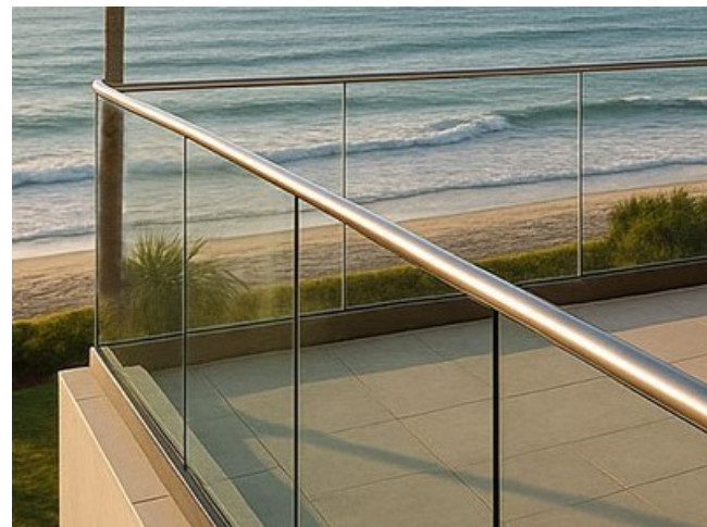
GL-03: CLEAR, LAMINATED GUARDRAIL ON SHOE
