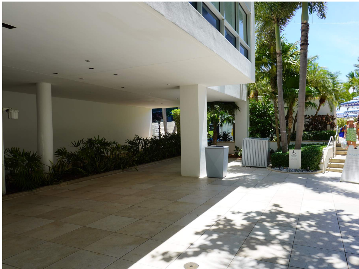
3. VIEW OF EXISTING AREA WHERE RESTROOMS WILL EXPAND
