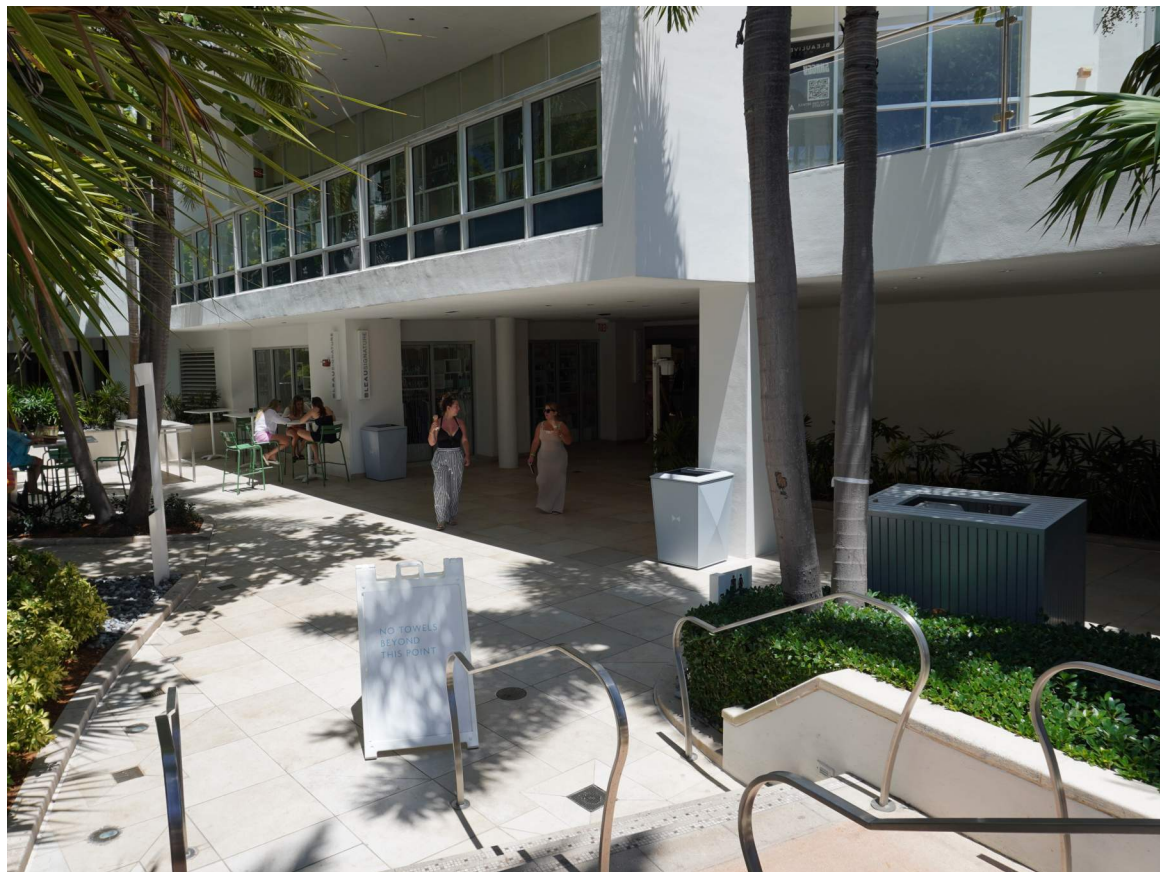
1. VIEW OF EXISTING RESTROOMS
