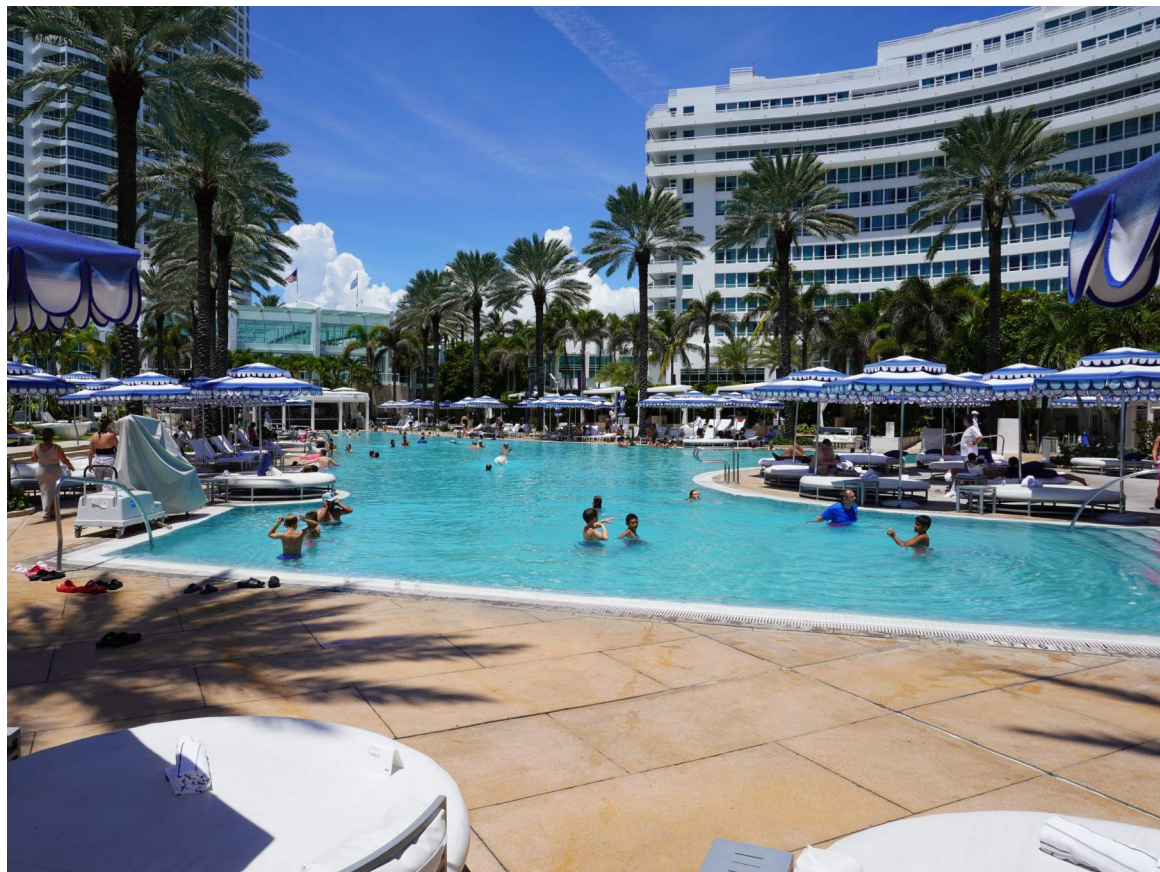
1. VIEW OF EXISTING BOWTIE POOL
