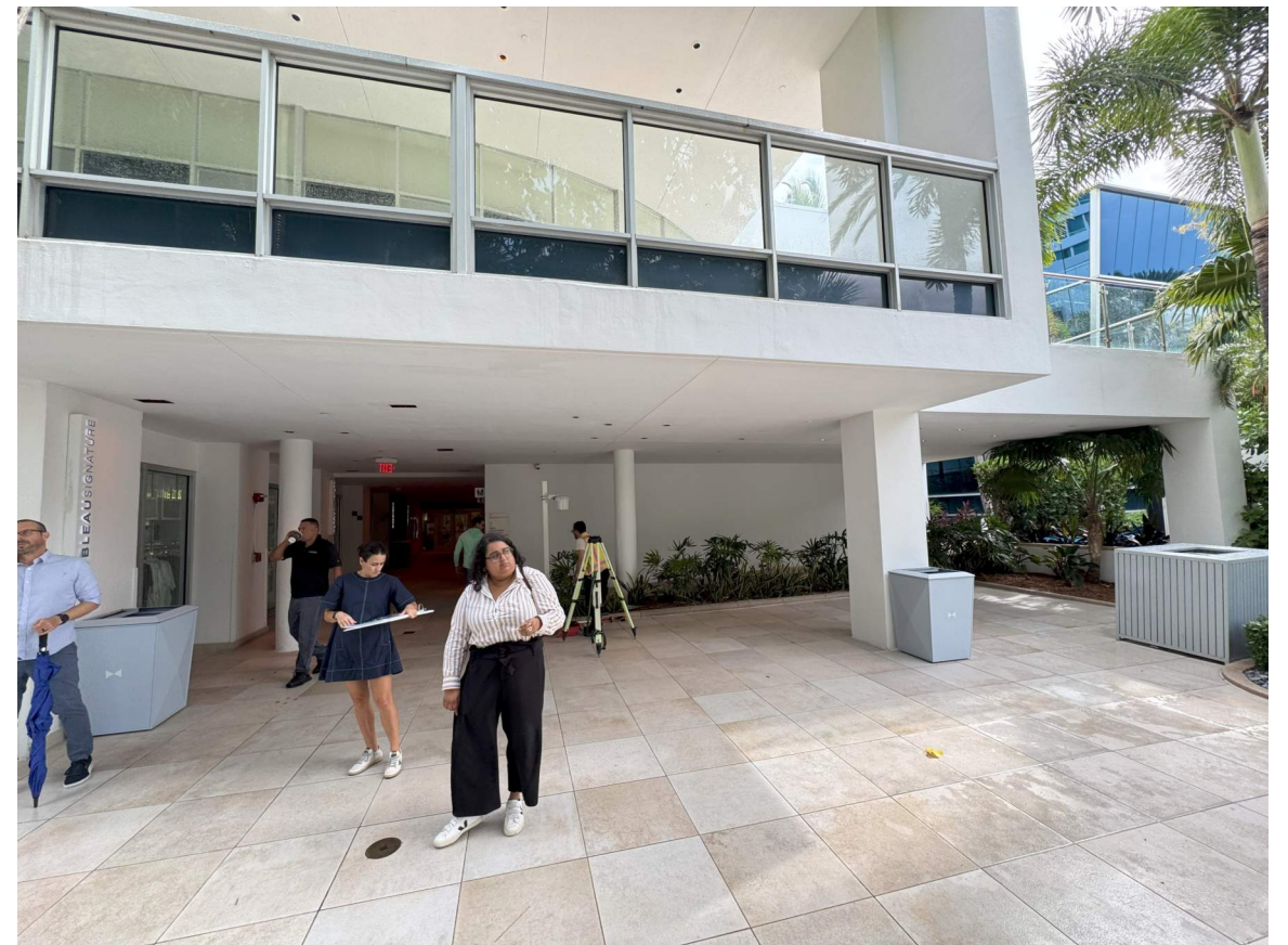
2. VIEW OF EXISTING RESTROOMS
