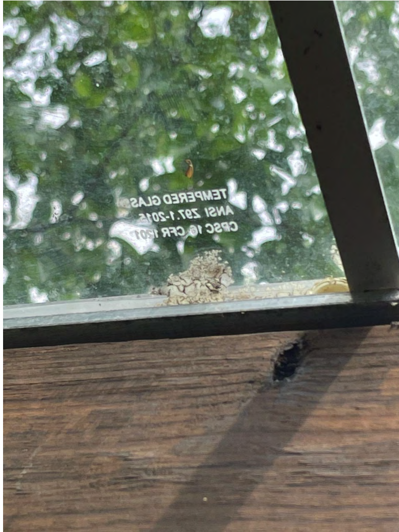
1 Tempered Glass Trellis Cover on Pressure Treated Wood Framing
