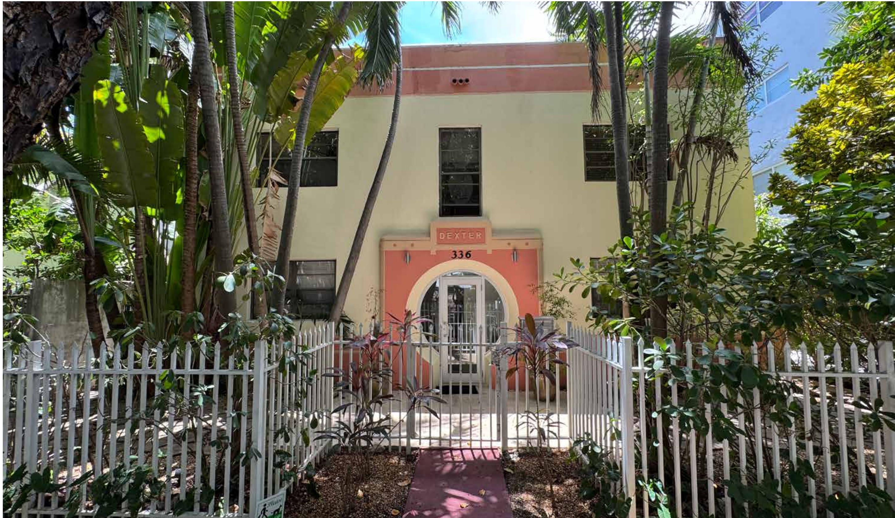
Existing Front (East) Façade
