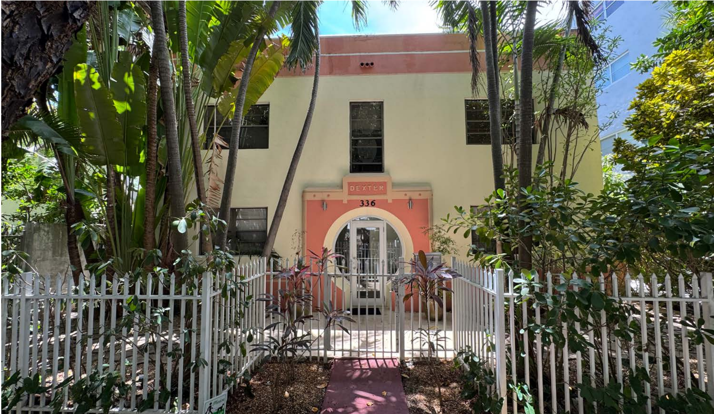
Existing Front (East) Façade
