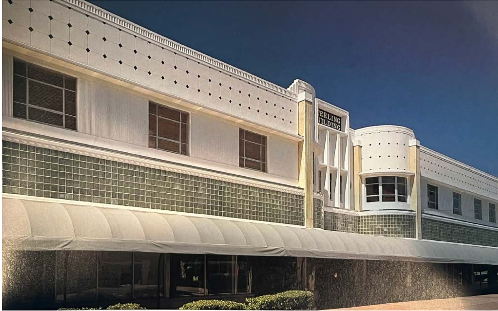
Sterling Building 1925 Miami Beach, Florida
