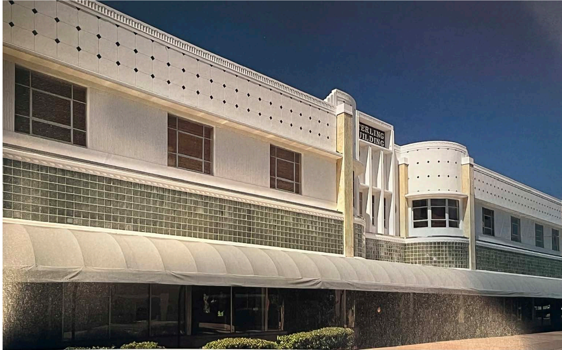
Sterling Building 1925 Miami Beach, Florida
