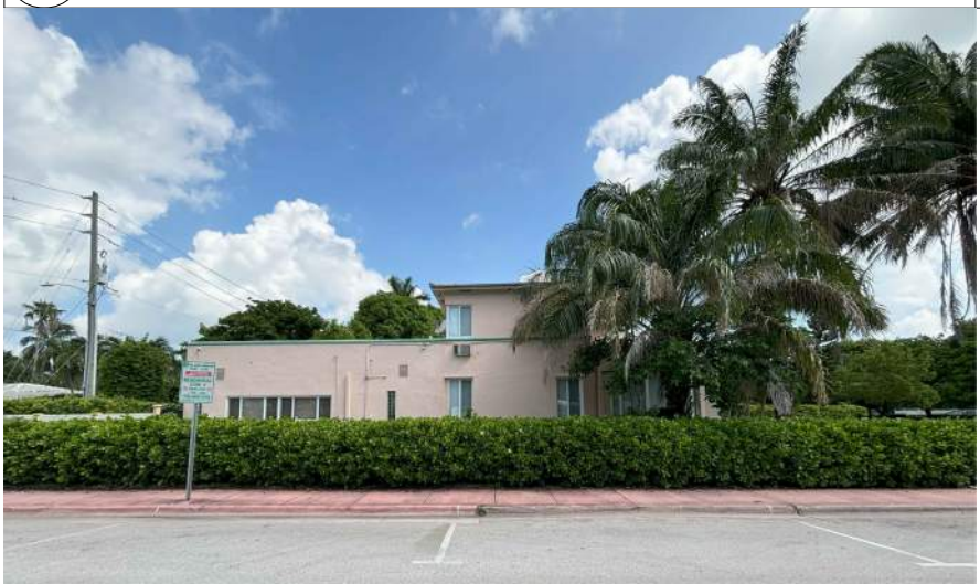
③ SITE PHOTO 3 (12TH STREET SIDE VIEW) A-0.3A Scale: NT5
