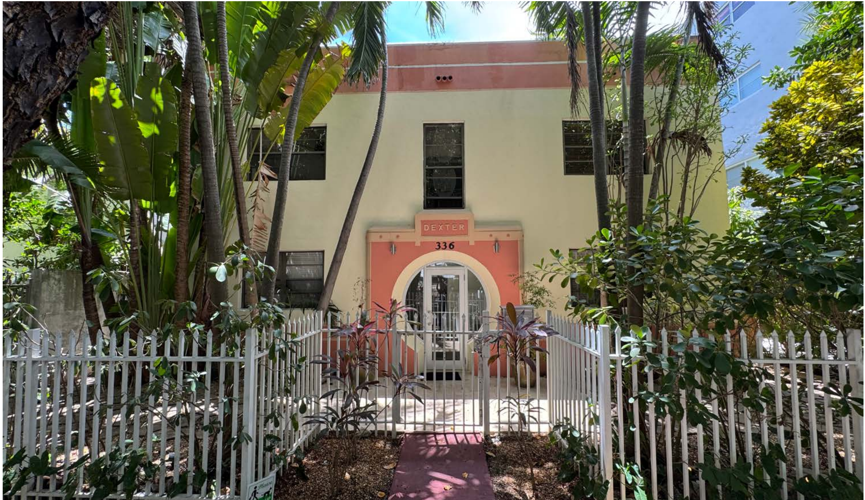
Existing Front (East) Façade
