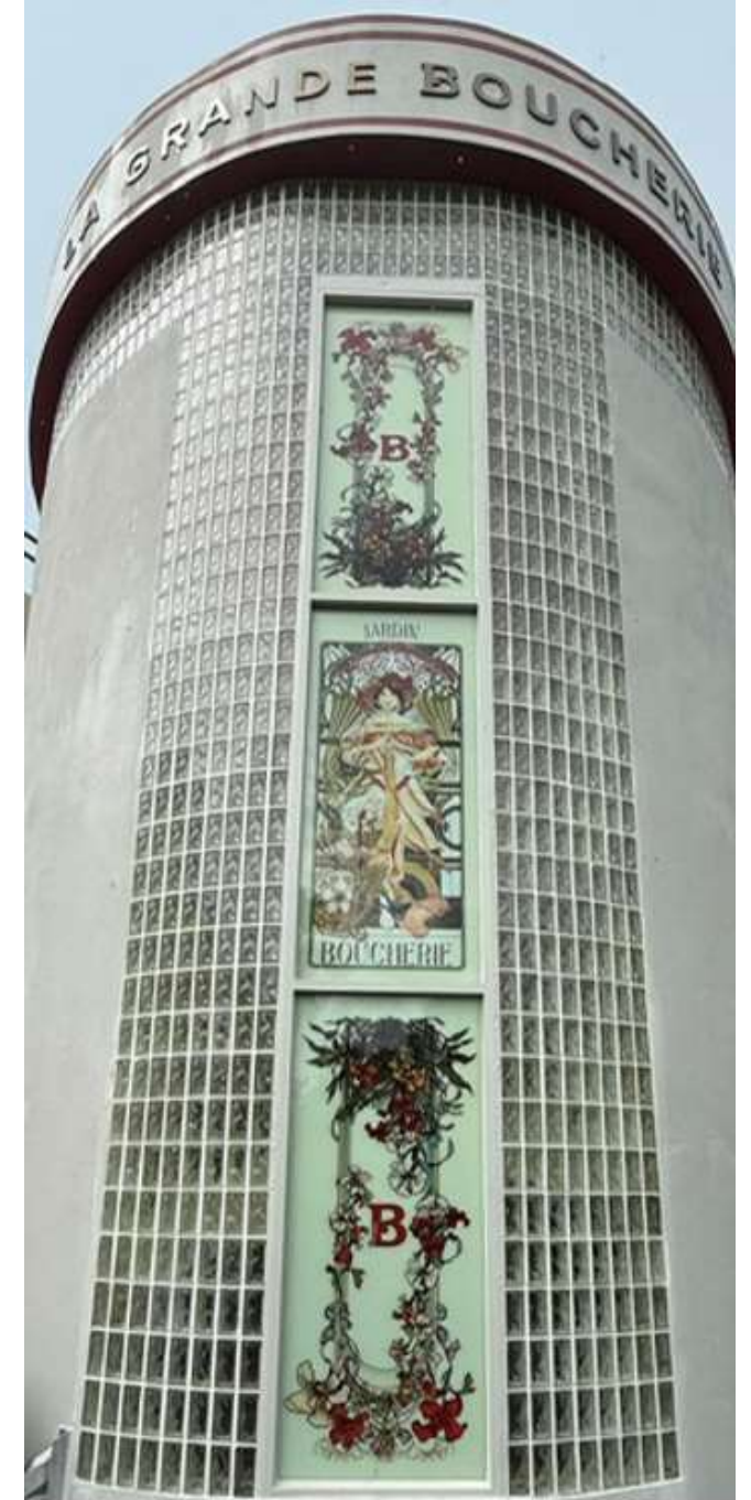
All 3 panels (view from roof)
