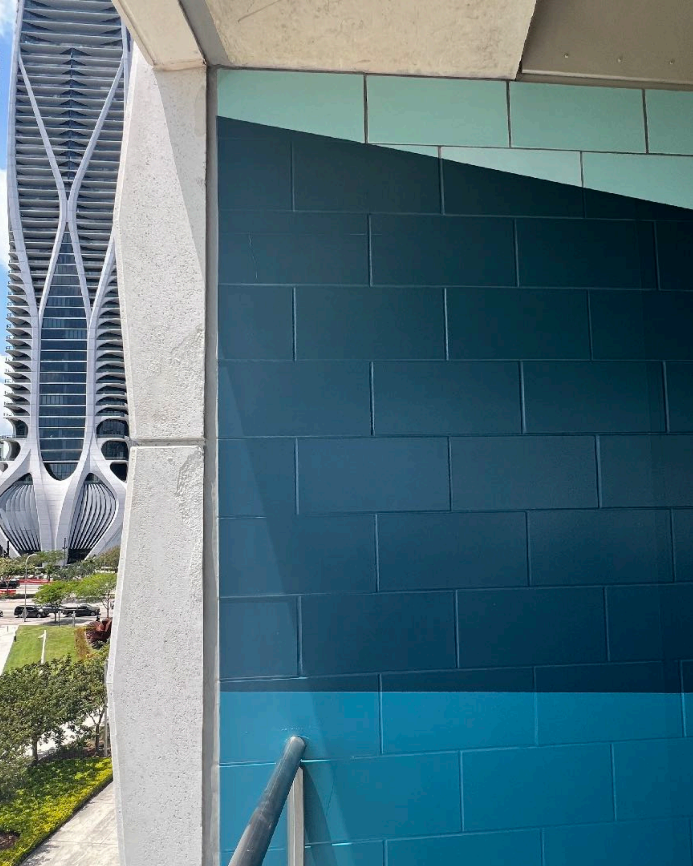
Concrete Vinyl exposed to outside weather after three years at Frost Science Museum
