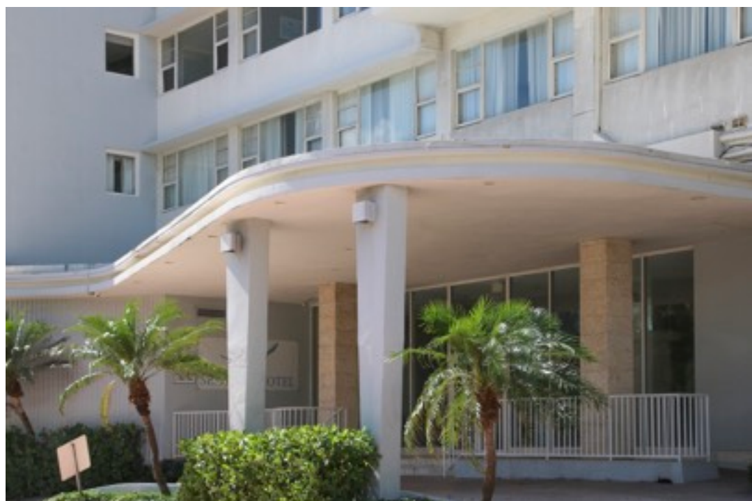
BELOW: PORTE-COCHERE WITH TWO OUTSIDE CONCRETE COLUMNS AND TWO INNER COLUMNS WHICH ARE CLAD WITH FIELDSTONE.
