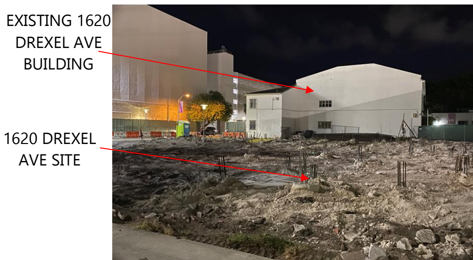
Figure 2 - Street View of 1620 Drexel Ave. The proposed building site is demolished.
