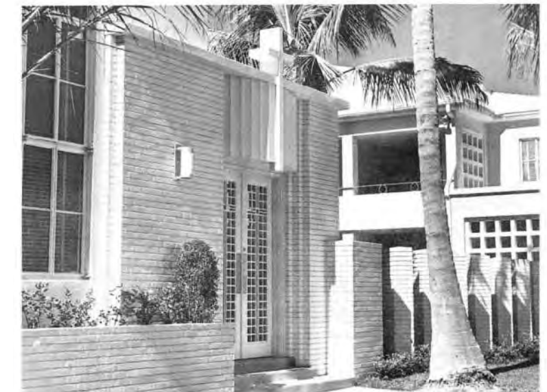
IMAGE OF COMPLETED ADDITION
