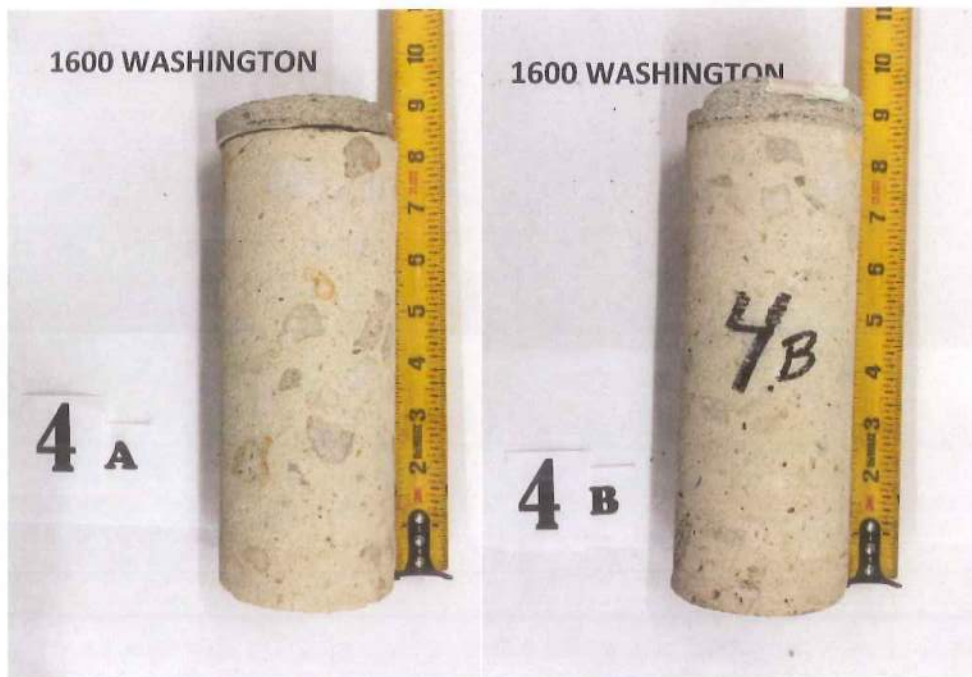
Figure 5: Photograph of Core Samples Level 2 (Compression/Chloride/Carbonation Samples)
