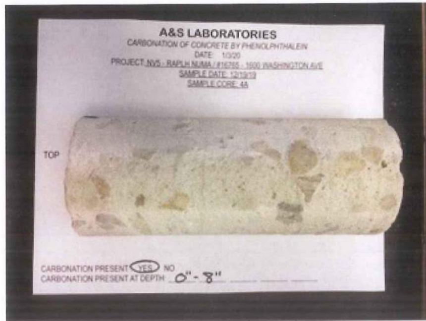
Figure 11: Photograph Core Sample No. 4A: Level 2 Column
