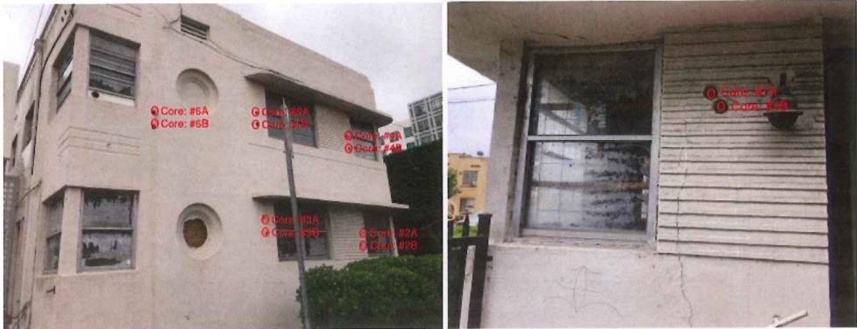
Figure 1: 1600 Washington Ave. - Approximate Concrete Core Locations
