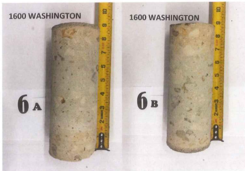
Figure 7: Photograph of Core Samples Level 2 (Compression/Chloride/Carbonation Samples)
