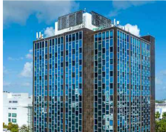
407 LINCOLN ROAD OFFICE TOWER EXISTING THIRTEEN STORY BUILDING
