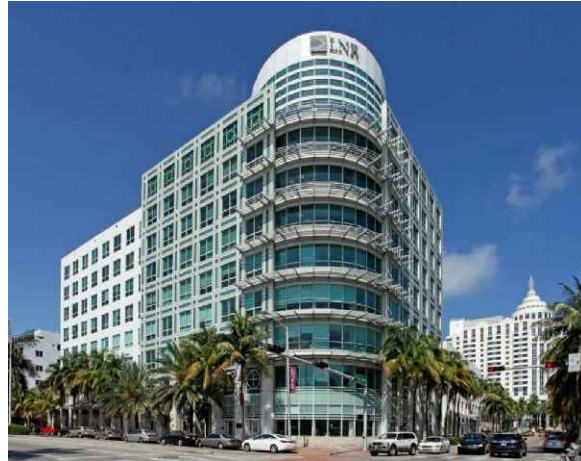
1601 WASHINGTON AVE LNR PARTNERS HEADQUARTERS EXISTING EIGHT STORY BUILDING
