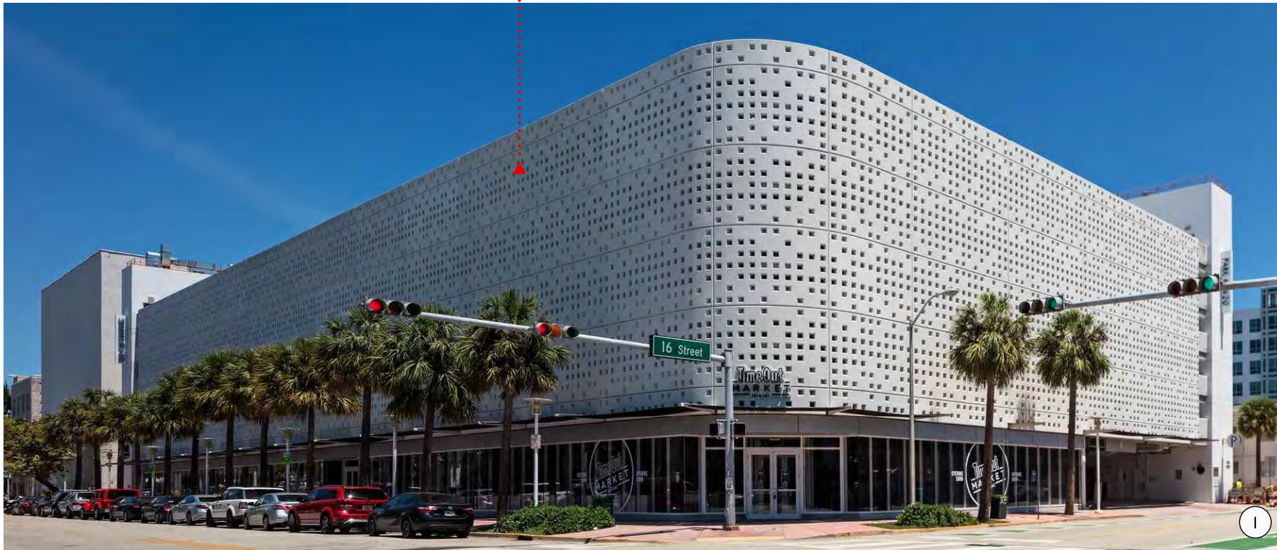
1601 DREXEL AVE EXISTING GARAGE BUILDING TO REMAIN
