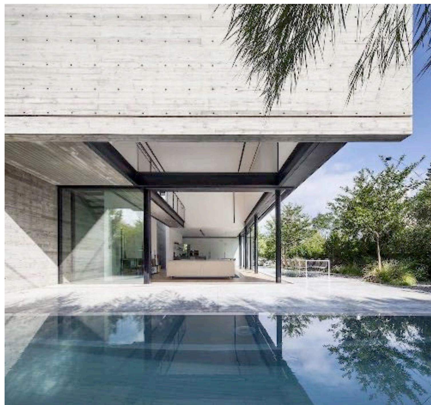
SLIDING DOORS & OFF-FORM CONCRETE WALLS
