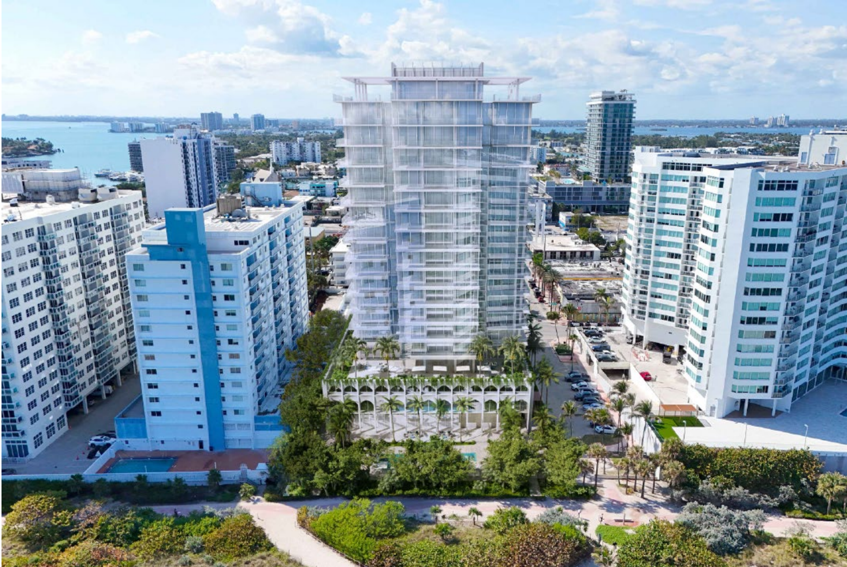
HPB25-0652: 6979 & 6985 Collins Avenue September 16, 2025
