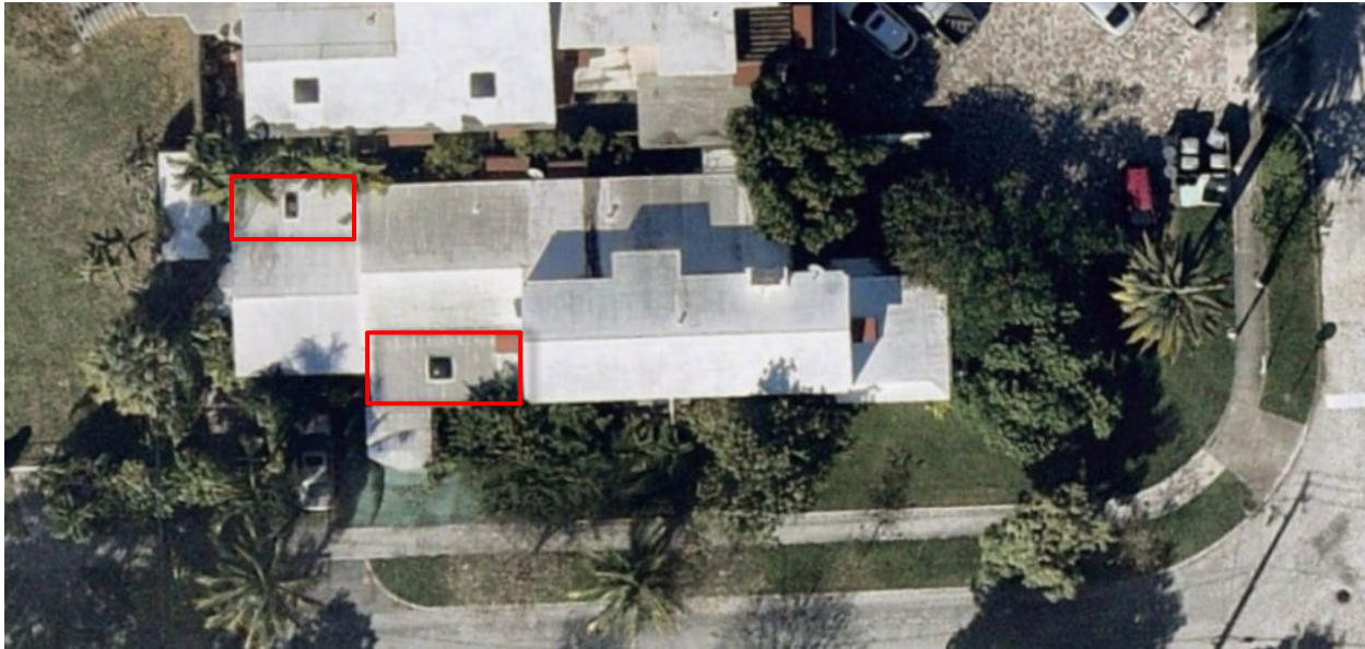
Aerial photograph, 2020 (unpermitted additions outlined in red)
