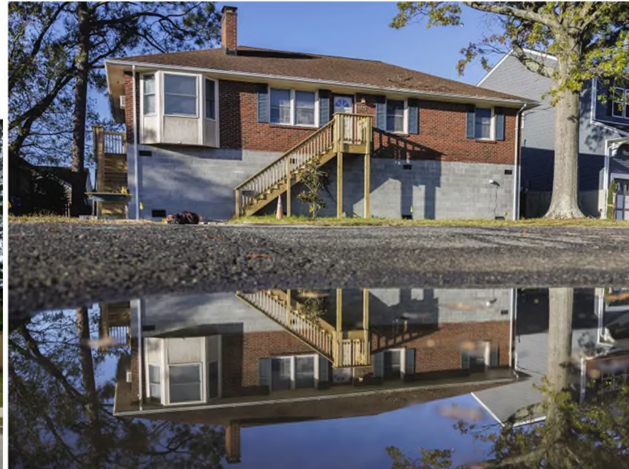
Photo By Sam Raising homes, which involves lifting it off the ground and building a new higher foundation below it, is one way homeowners are protecting their properties from flooding. | Lathan Goumas/Virginia Sea Grant, CC BY-ND 4.0
