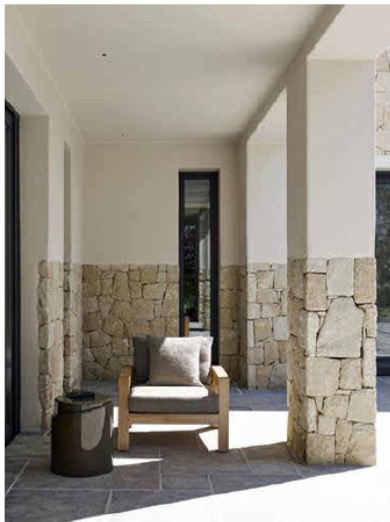
WHITE STUCCO, CORAL ROCK REVEALS AND DETAIL
