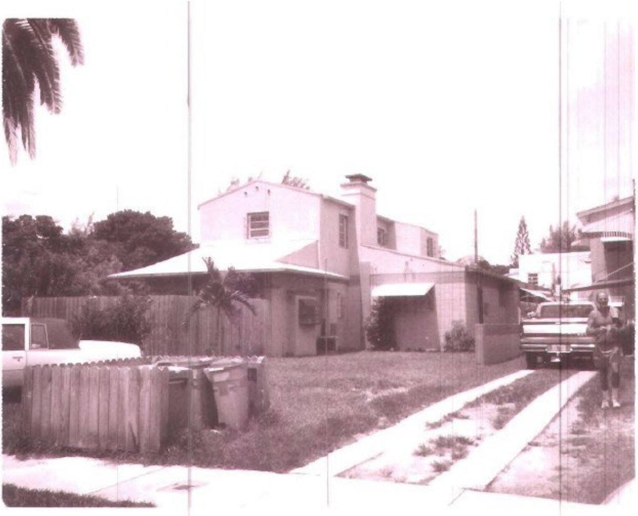
1969 view facing SW on Michigan Ave
