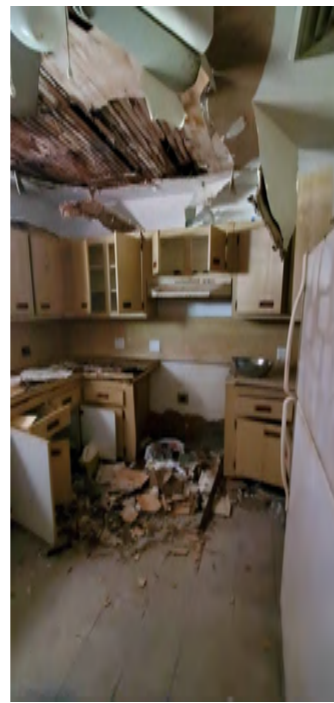
3 INTERIOR OF HOUSE 2 1" = 20'-0"
