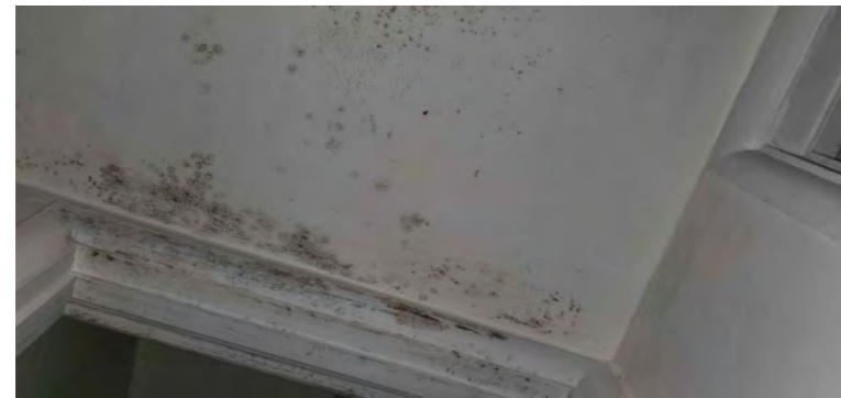
2 INTERIOR OF HOUSE 1 1" = 20'-0"
