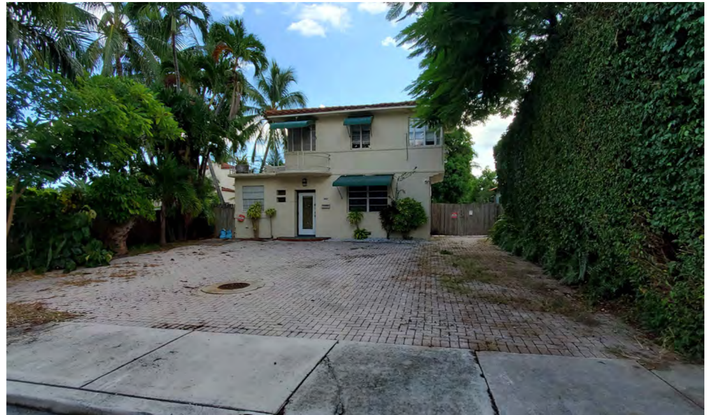
12 VIEW OF LOT 1827 FACING EAST 1 1/2" = 1'-0"
