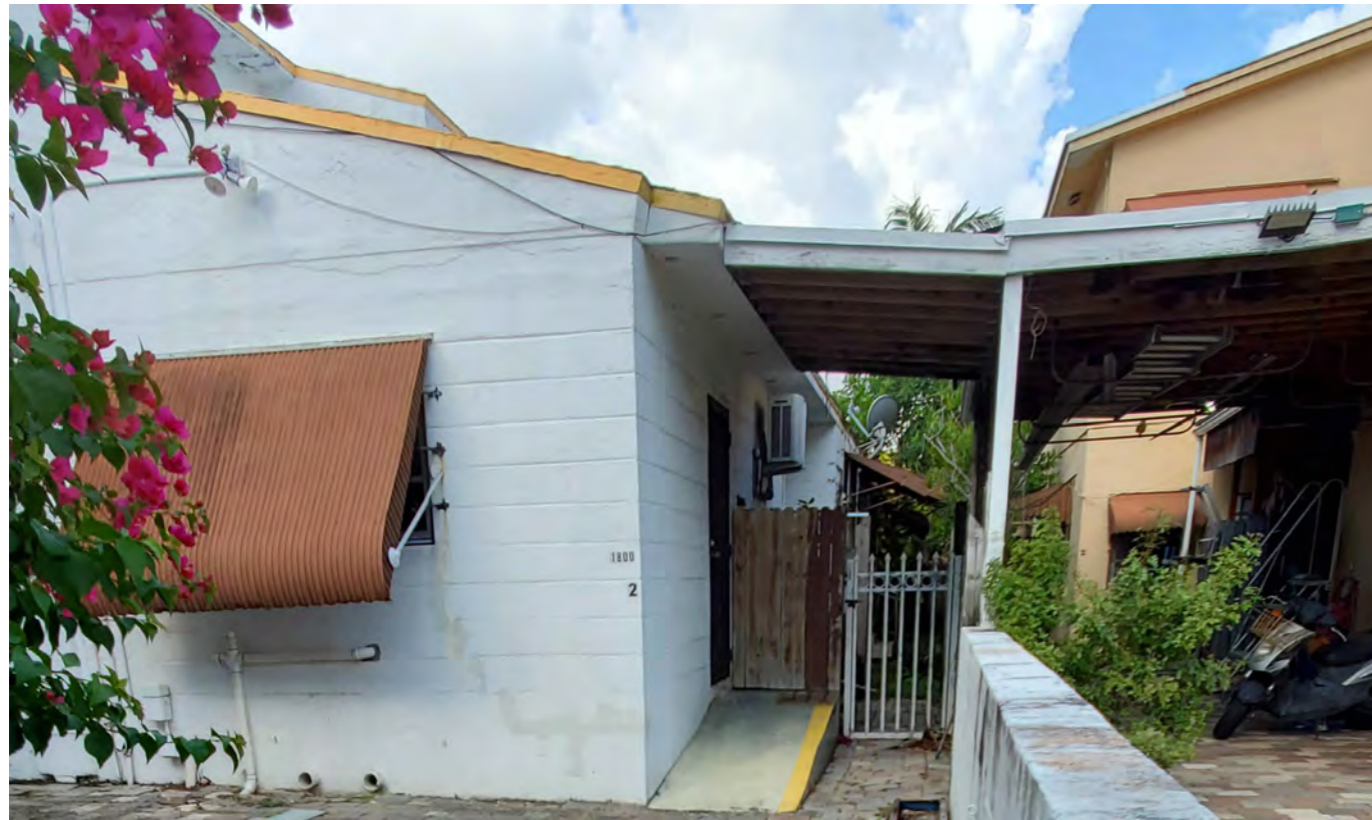
9 VIEW OF LOT 1800 FACING WEST 1 1/2" = 1'-0"
