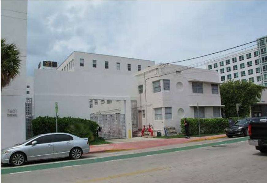
16th Street Frontage of 420 garage service yard and Laurel Apartments View looking North
