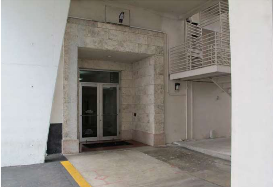
Rear (south) entrance to the Mercantile National Bank Building. View looking North.
