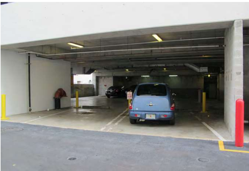
Base level of the 420 Garage. View looking south.
