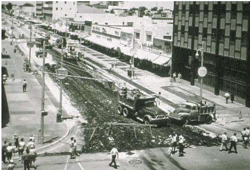
top: Aerial View of Lincoln Road Mall under construction. Date unknown. Courtesy of The Miami Herald
