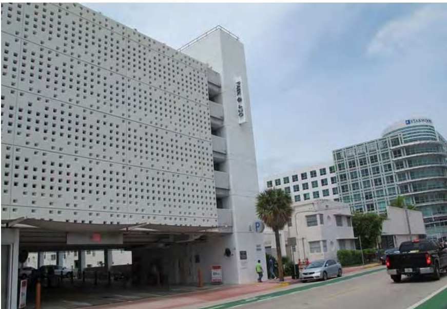
16th Street Frontage of 420 Garage View looking East
