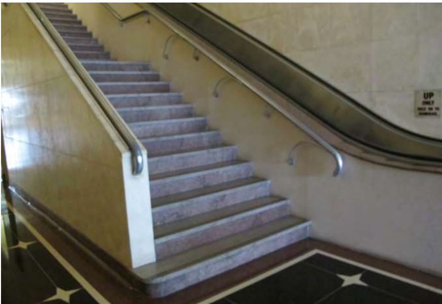
Mercantile National Bank Building. Detail of main stair.
