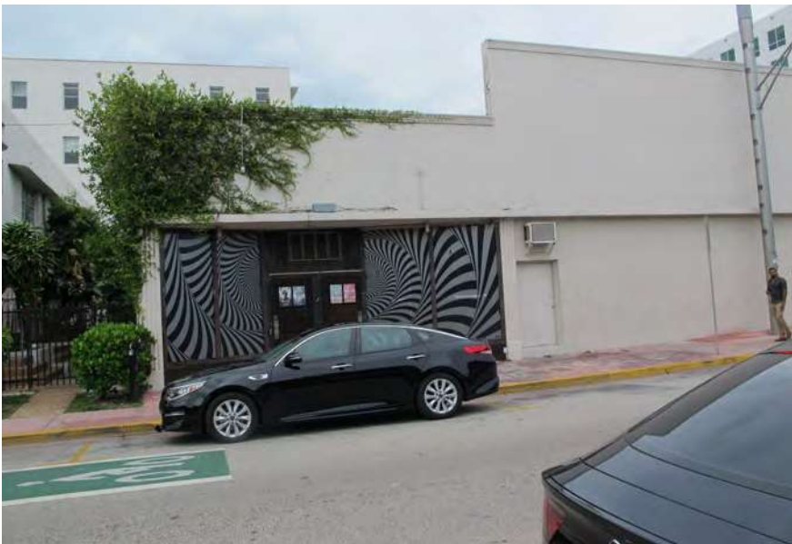
1600 Washington Avenue, 16th Street side 423, 16th Street, view looking north
