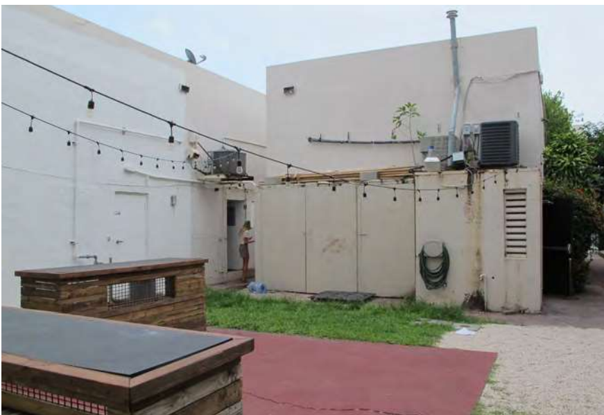
Rear courtyard of 423 16th Street View looking south
