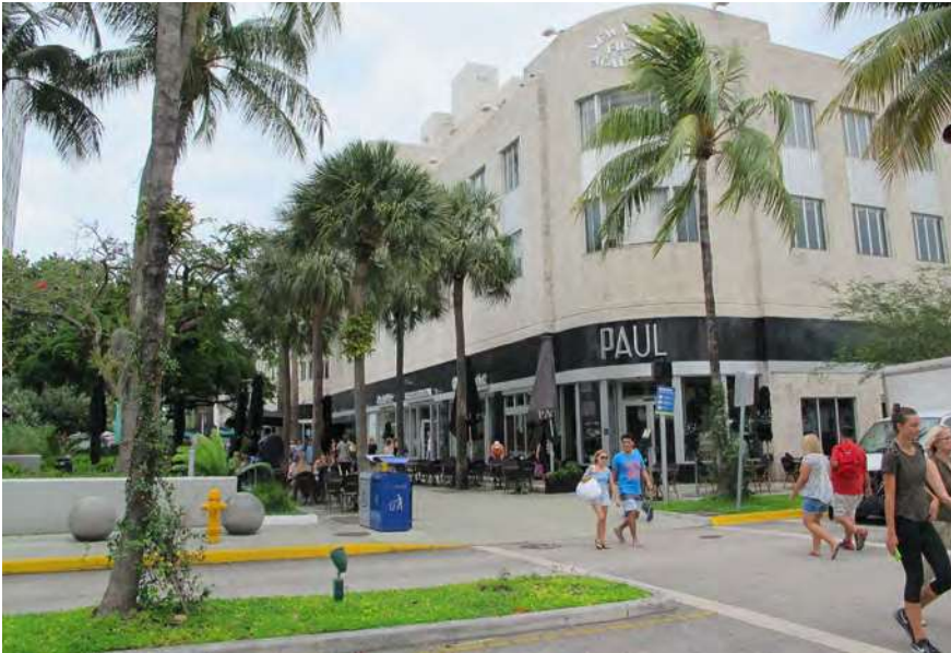
Mercantile National Bank Building Lincoln Road/Drexel Avenue facade. View looking east.
