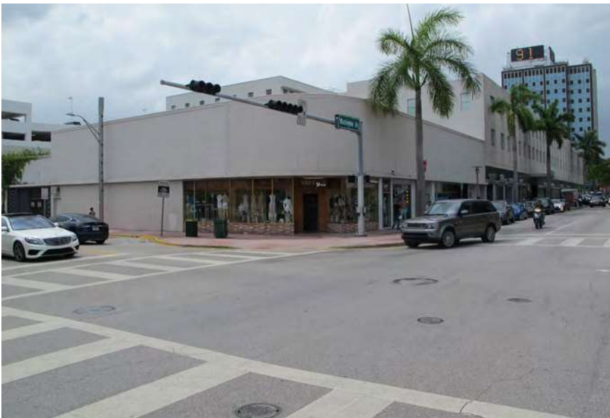
Corner of 1600 Washington Avenue Building. View looking north along Washington Avenue
