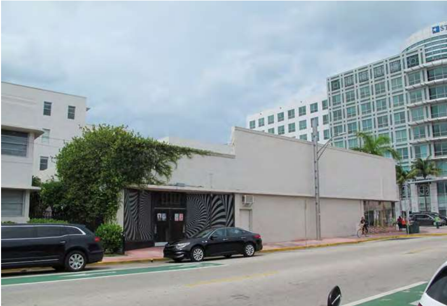
South facade at 1600 Washington Avenue Building. View looking northeast.
