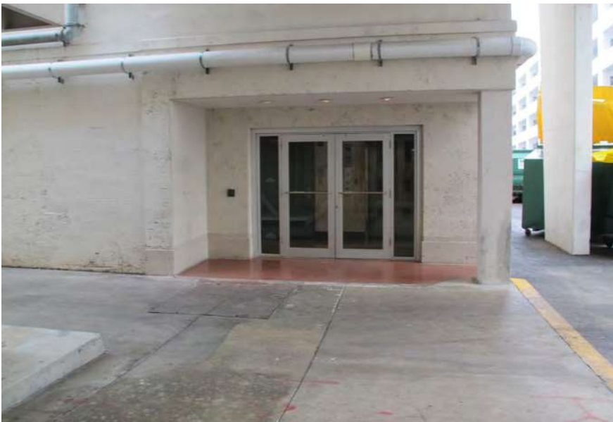
Rear (west) entrance to the Washington Avenue Annex Building. View looking South.
