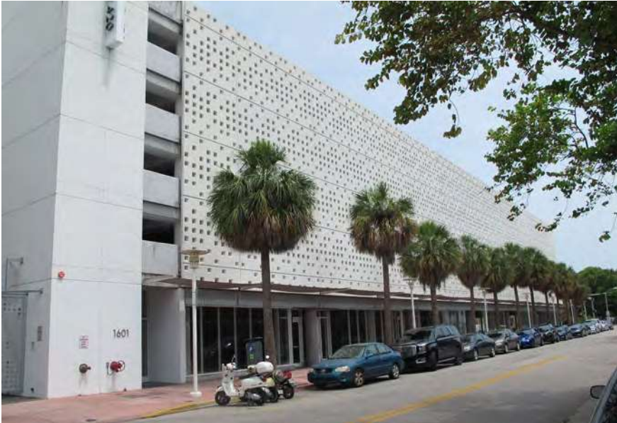
Drexel Avenue Frontage View Looking South
