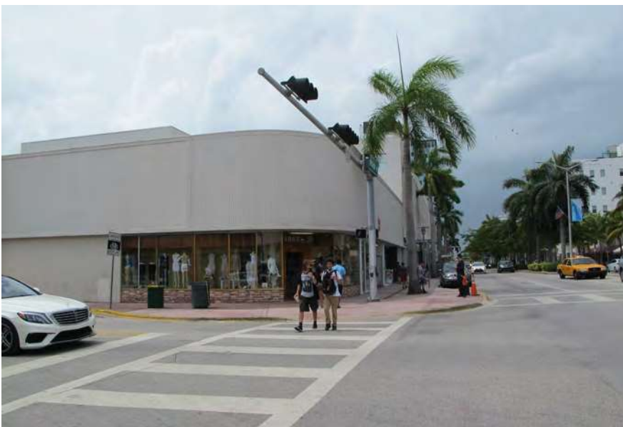
Corner and east facade of Washing- ton Avenue Building. View looking Northeast.
