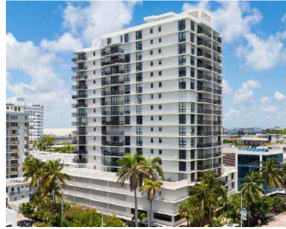
1800 COLLINS AVENUE TOWER 1800 EXISTING NINETEEN STORY BUILDING
