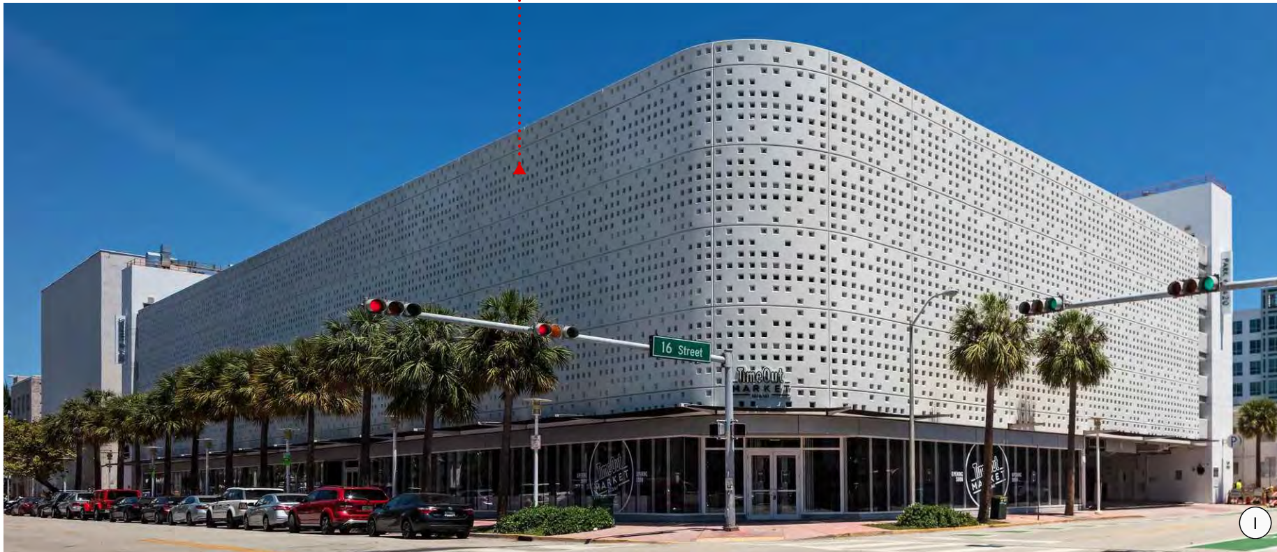
1601 DREXEL AVE EXISTING GARAGE BUILDING TO REMAIN
