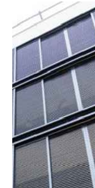
ALUMINUM 'Z' LOUVERS ATTACHED THE BUILDING FACADE
