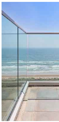
TEMPERED SAFETY GLASS GUARDRAIL AT ROOFTOP DECK
