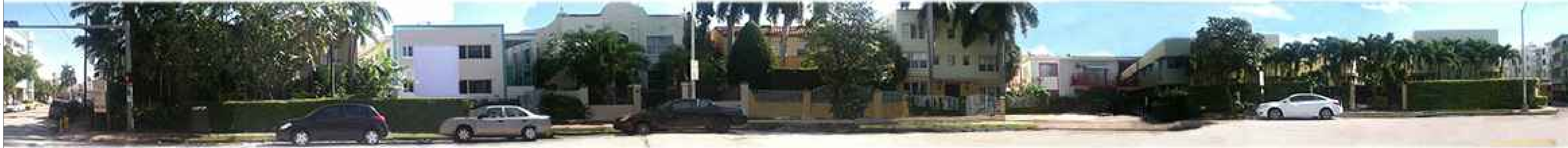
2 PANORAMIC OF BLOCK IN FRONT OF SITE
