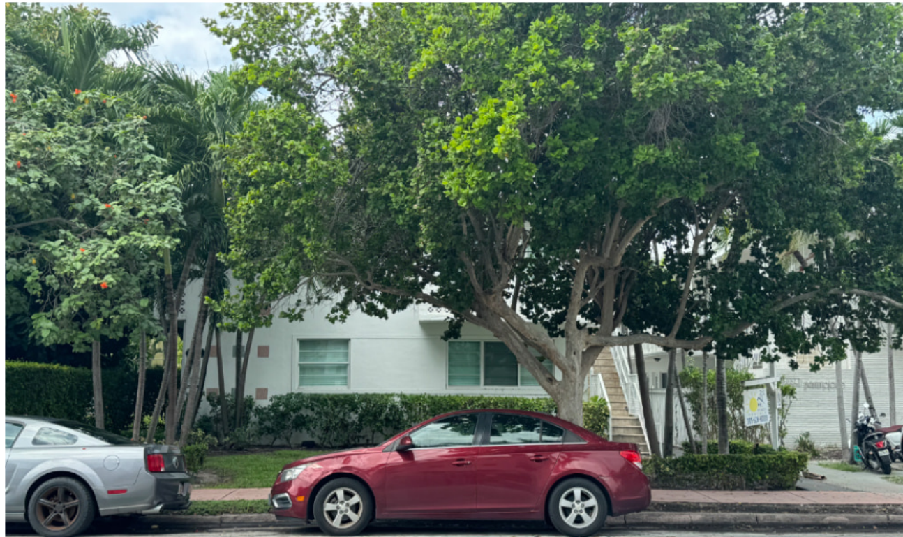
3 1026 PENNSYLVANIA AVE EXISTING TWO-STORY BUILDING
