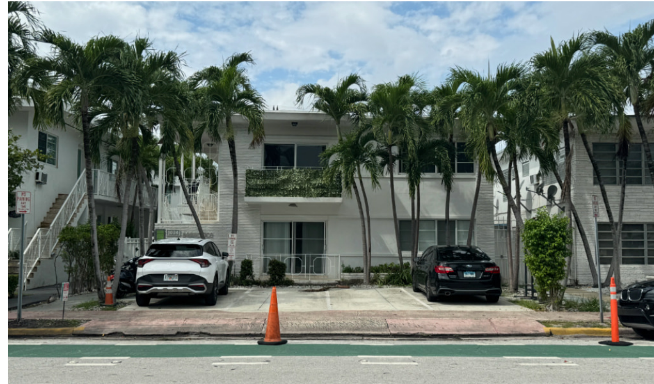
2 1034 PENNSYLVANIA AVE EXISTING ONE-STORY BUILDING
