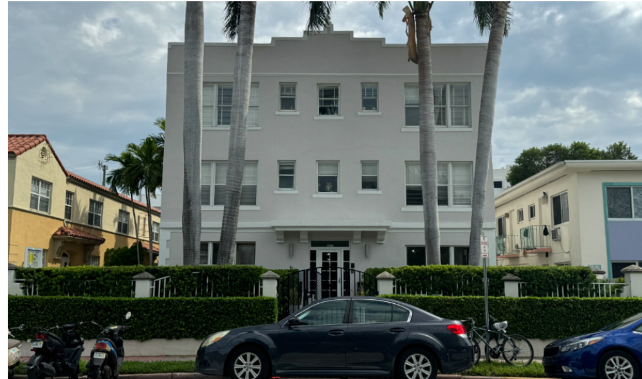
10 1027 PENNSYLVANIA AVE EXISTING THREE-STORY BUILDING
