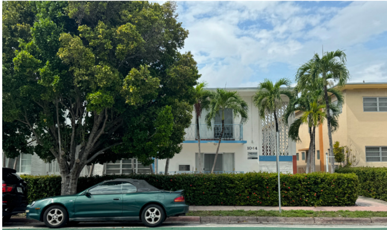
1 1044 PENNSYLVANIA AVE EXISTING TWO-STORY BUILDING
