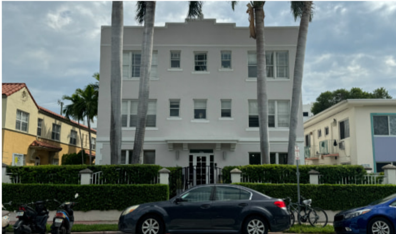
10 1027 PENNSYLVANIA AVE EXISTING THREE-STORY BUILDING
