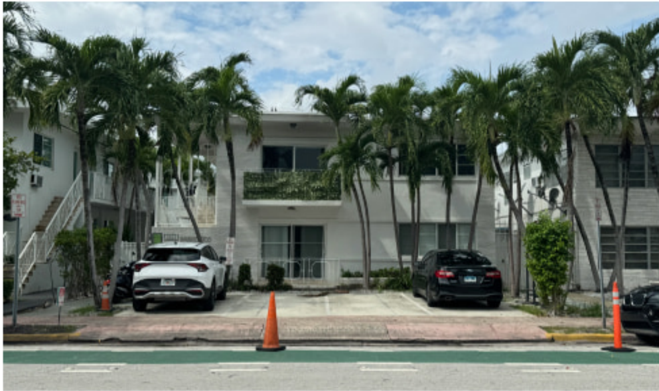
2 1034 PENNSYLVANIA AVE EXISTING ONE-STORY BUILDING
