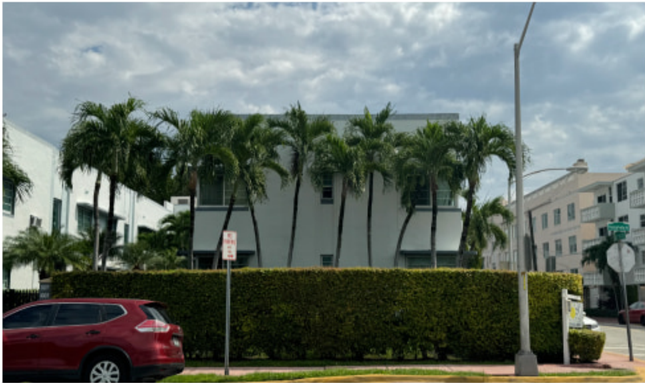
7 1003 PENNSYLVANIA AVE EXISTING TWO-STORY BUILDING
