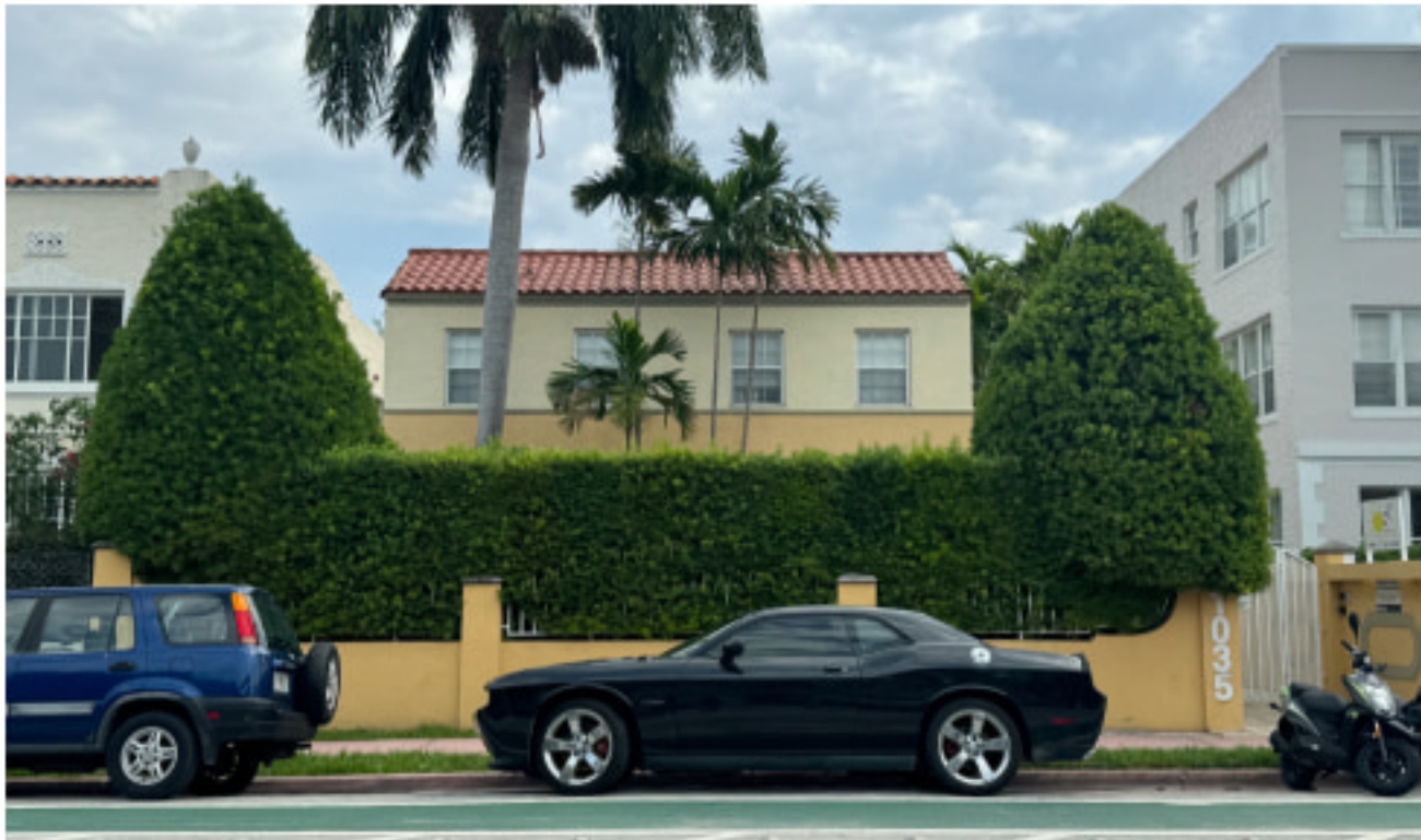
11 1035 PENNSYLVANIA AVE EXISTING TWO-STORY BUILDING
