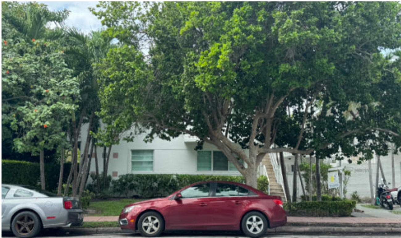
3 1026 PENNSYLVANIA AVE EXISTING TWO-STORY BUILDING
