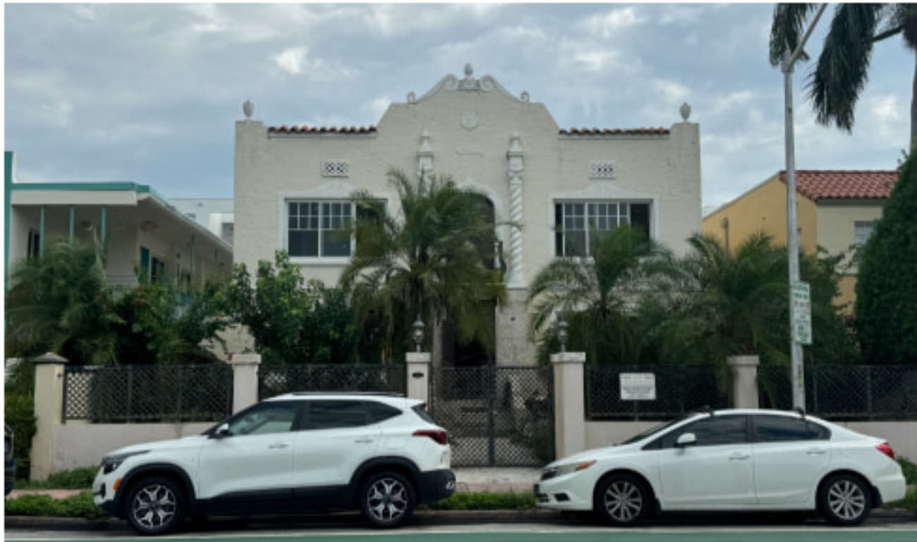
12 1045 PENNSYLVANIA AVE EXISTING TWO-STORY BUILDING
