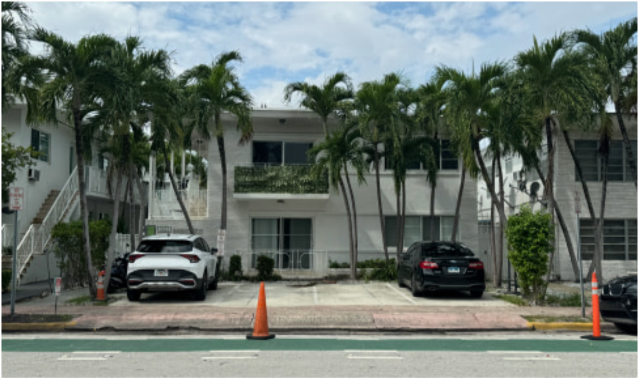
2 1034 PENNSYLVANIA AVE EXISTING ONE-STORY BUILDING
