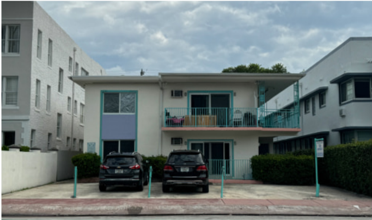
9 1023 PENNSYLVANIA AVE EXISTING TWO-STORY BUILDING
