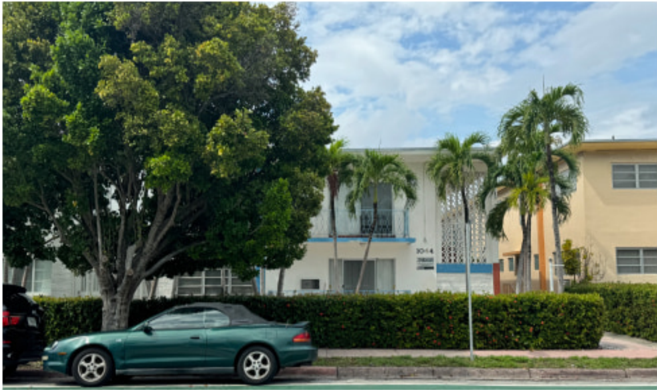
1 1044 PENNSYLVANIA AVE EXISTING TWO-STORY BUILDING
